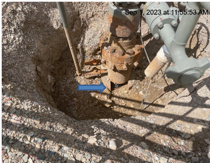
Photo # 8069 MCU 26-4A well, gas is bubbling up from conductor
