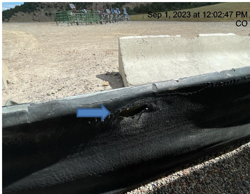
Photo # 8087 Hole in secondary containment liner/liner needs maintenance
