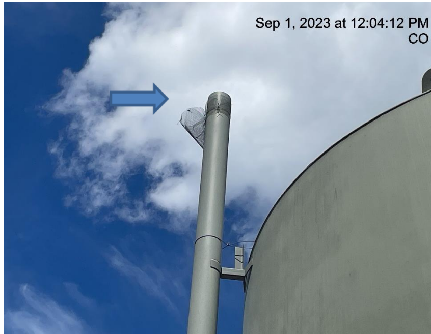
Photo # 8100 Bird protection on 500 bbl heated condensate tank needs maintenance
