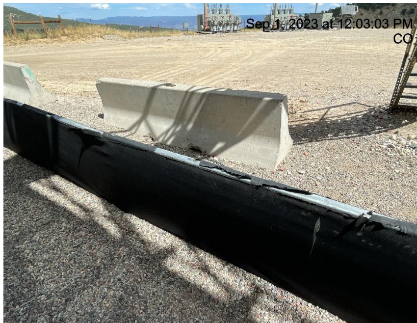
Photo # 8089 Liner needs maintenance
