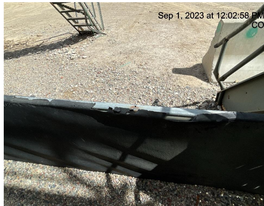
Photo # 8088 Liner needs maintenance
