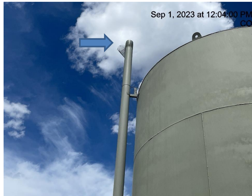
Photo # 8097 Bird protection on 500 bbl heated condensate tank needs maintenance
