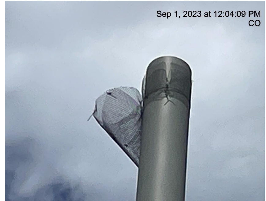
Photo # 8101 Bird protection on 500 bbl heated condensate tank needs maintenance
