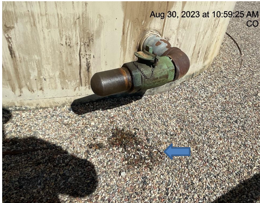
Photo # 7674 Stained gravel in secondary containment
