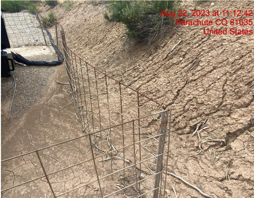
Insufficient Erosion Control – Photo #06039
