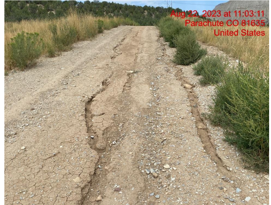
Rill Erosion Cutting Through Access Road – Photo #06027
