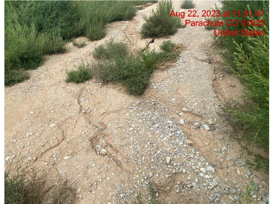
Rill Erosion Cutting Through Access Road – Photo #06025
