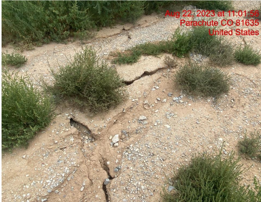
Rill Erosion Cutting Through Access Road – Photo #06026
