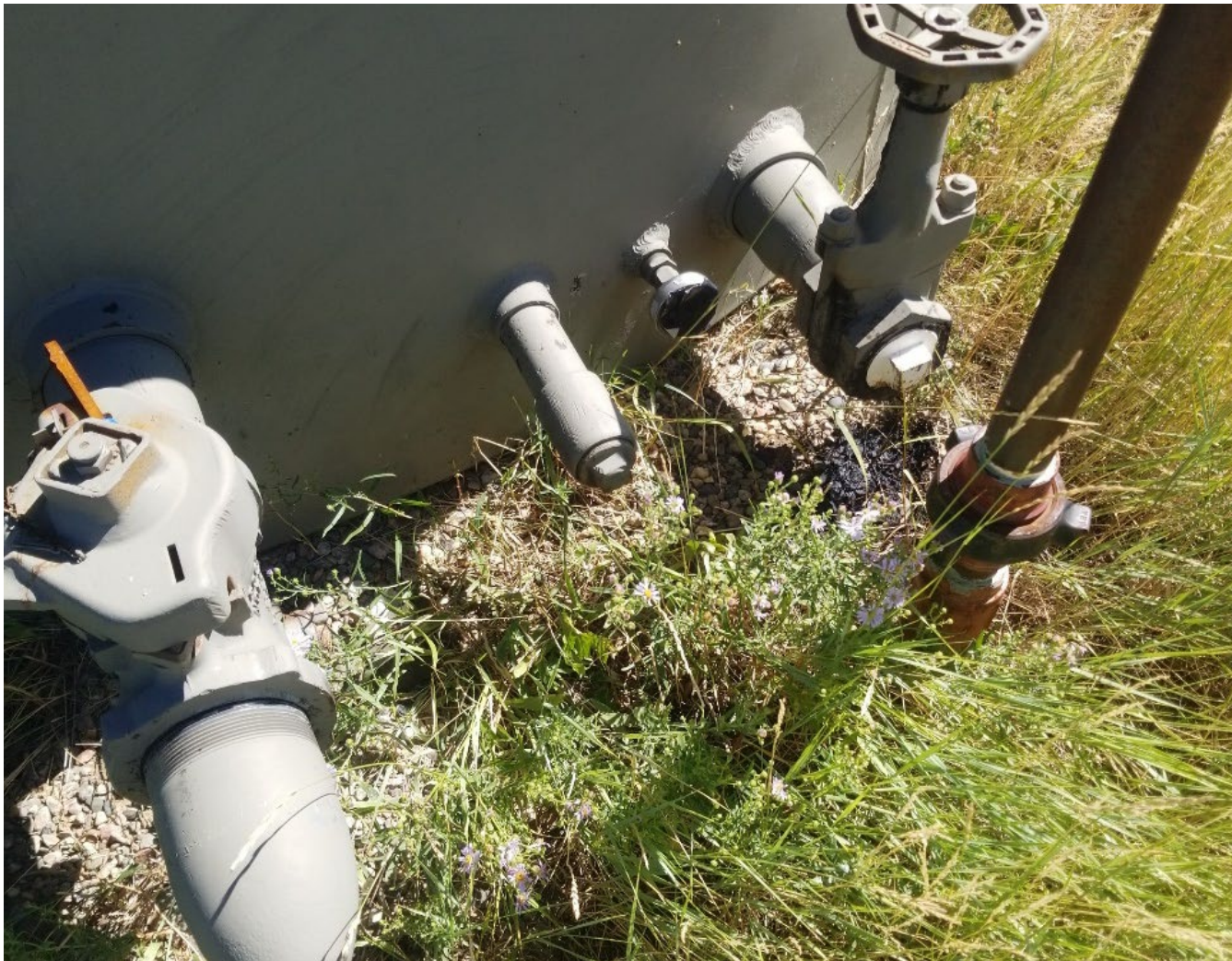
Photo #5 Back of tank. It appears that the blind plug in tank is PVC and is leaking.
