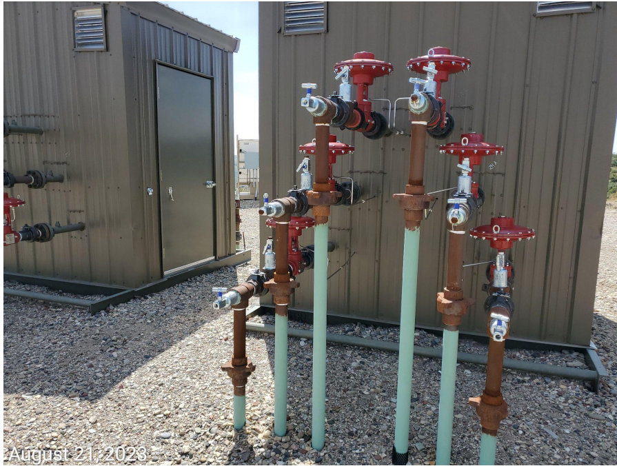
Photo 3: Example of uncapped lines observed at separators.
