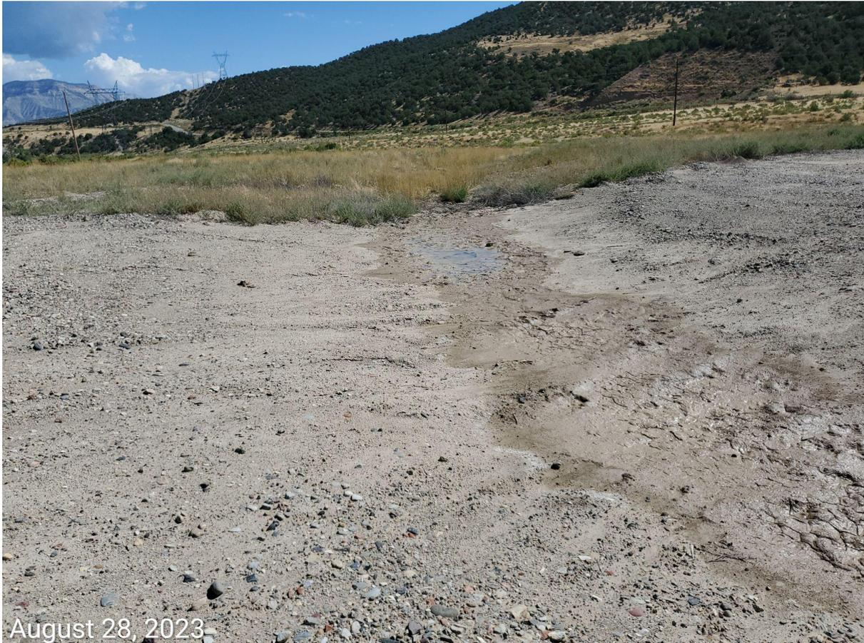
**Photo 7:** Photo shows contoured areas, on the north end of the working pad surface, that discharges stormwater into the interim areas to the north, and into the sediment trap observed within photos 5-6.
