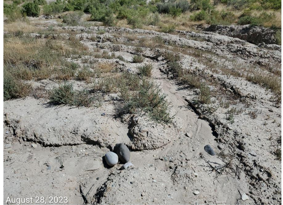
**Photo 4:** Photo shows erosion degradation due to stormwater runoff from the northeast corner of the working pad surface, behind the tank battery. BMPs to properly manage runoff remain inadequate.
