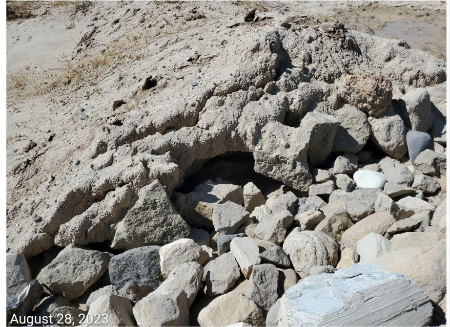
**Photo 5:** Photo taken from the sediment trap on the north east end of the Location. Photo shows outlet has not been installed per good engineering practices; rock armor has not been installed in conjunction with geotextile lining, resulting in degradation to the control.
