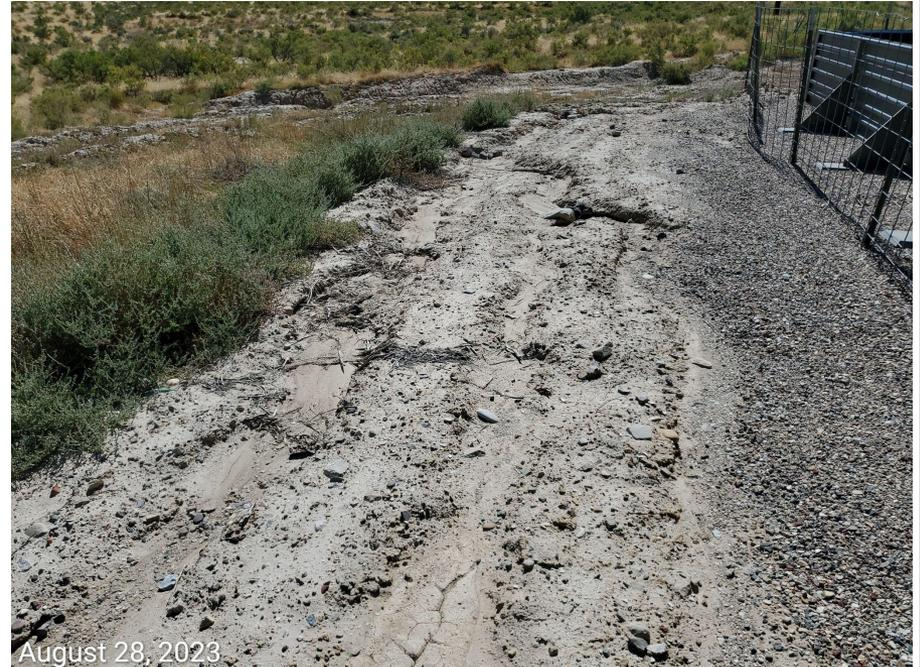
**Photo 3:** Photo taken from the northeast corner of the working pad surface. Photo shows control measures to allow for proper stormwater discharge remain missing or insufficient; erosion degradation has persisted.
