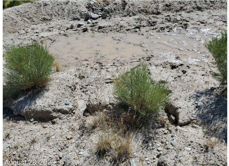
**Photo 6:** Photos shows sediment trap on the north east end of the Location has not been installed with a properly engineered inlet. Stormwater runoff from the pad is resulting in degradation to the control.
