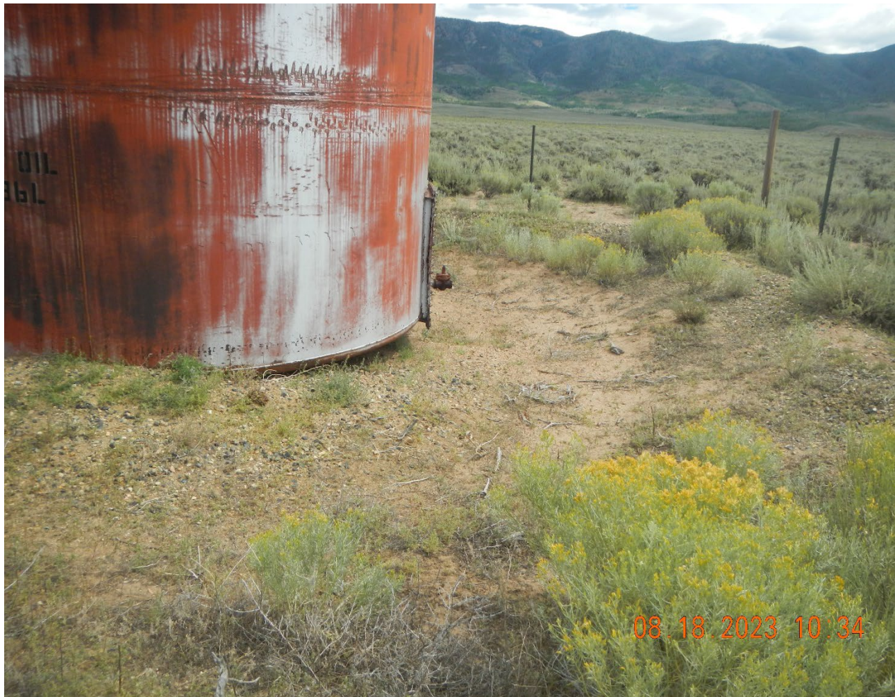
Photo #6 erosion under tank.
