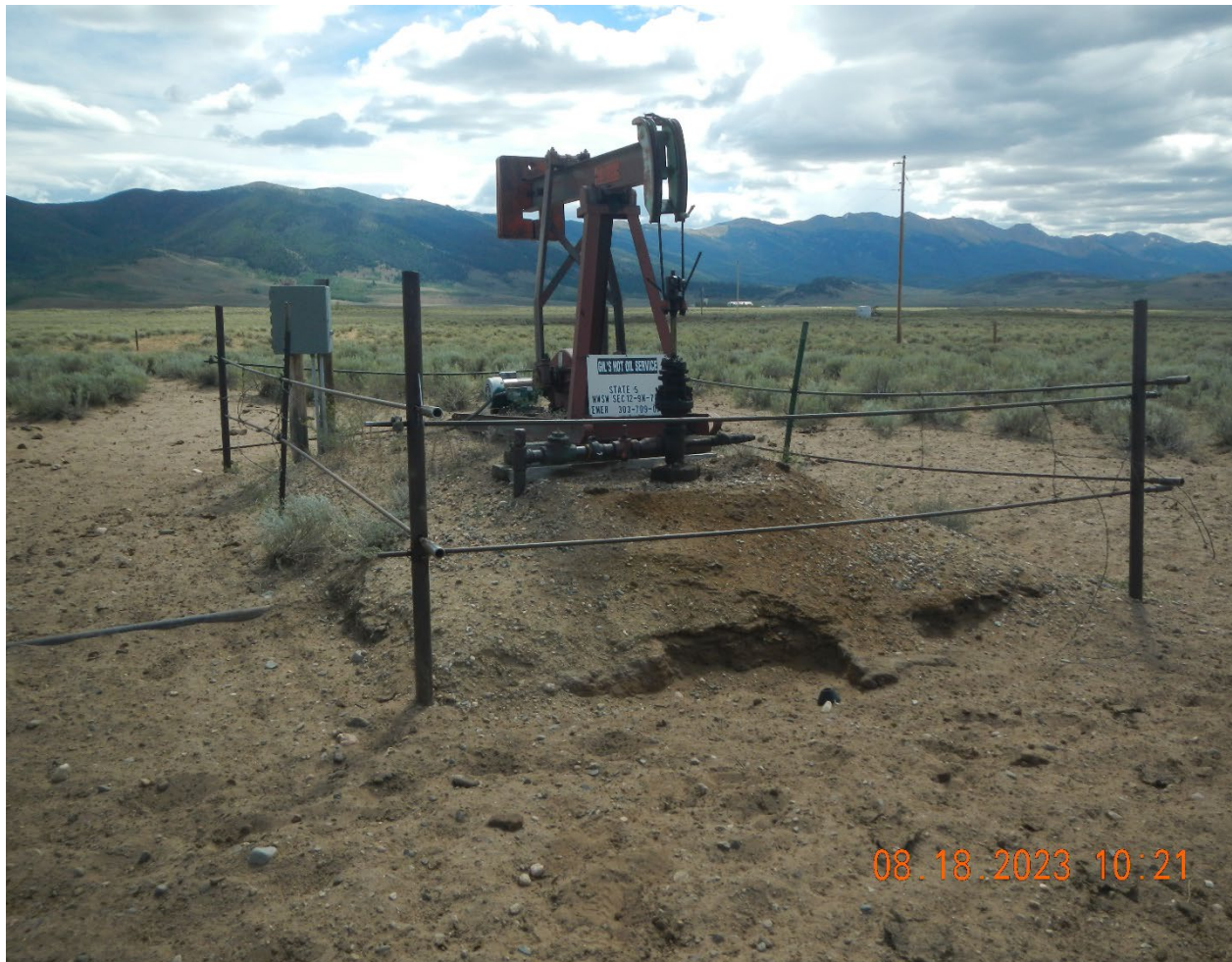
Photo #2 flowline on ground. Soil built up at wellhead had oil staining.
