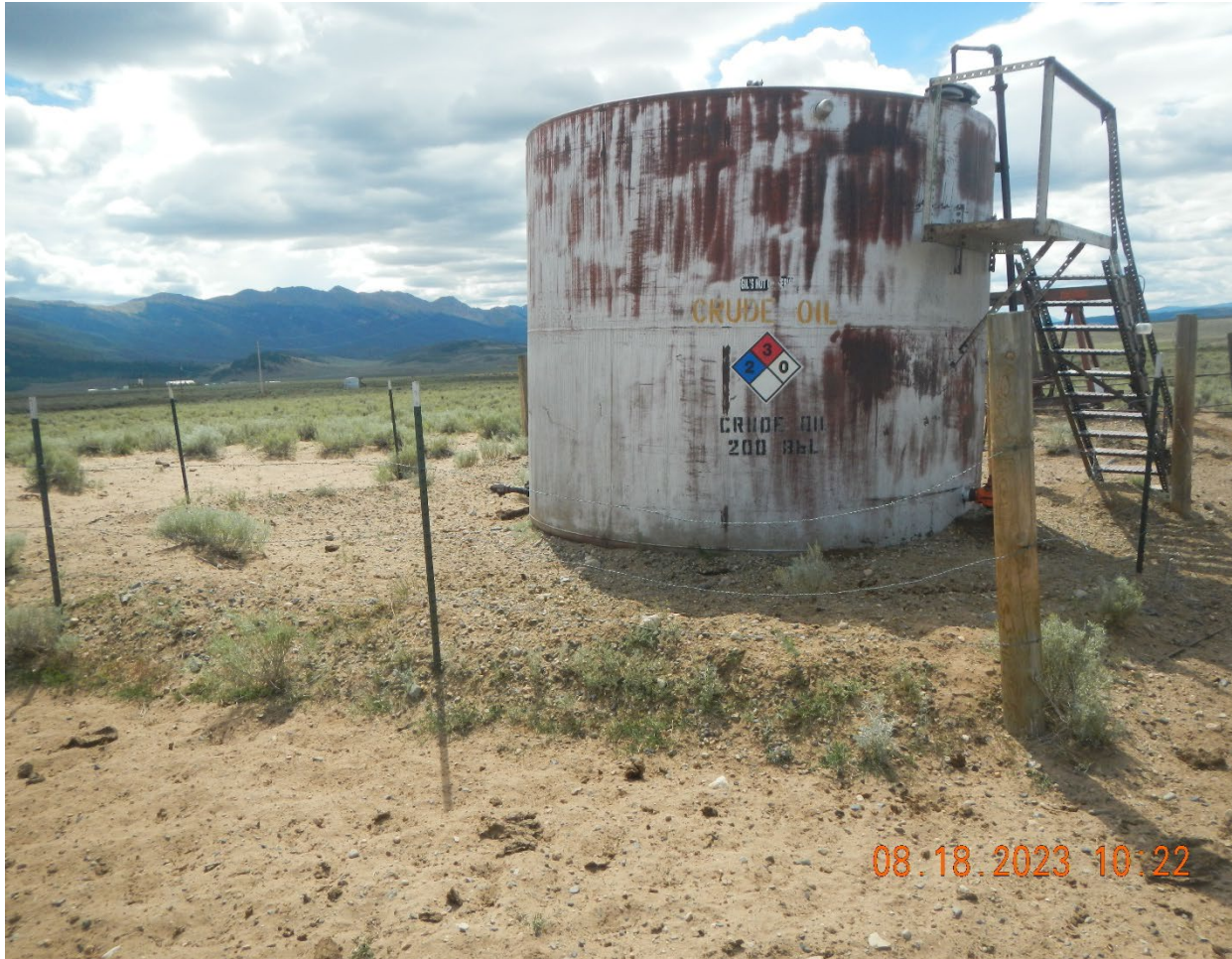
Photo #5 overview of Tank. Tank did not have adequate secondary containment. Soil type at tank is Sand.
