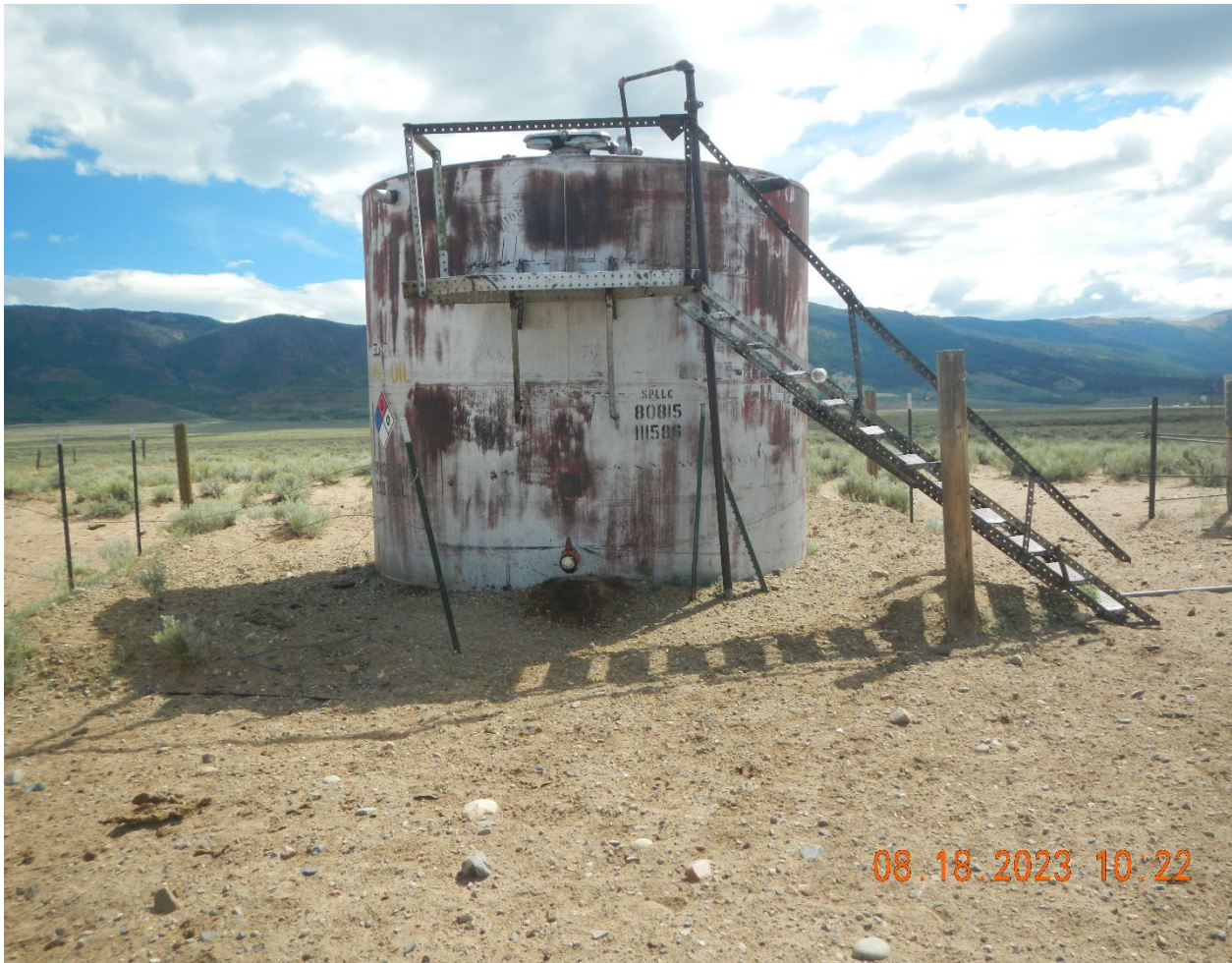
Photo #4 overview of Tank. Tank did not have adequate secondary containment. Soil type at tank is Sand.
