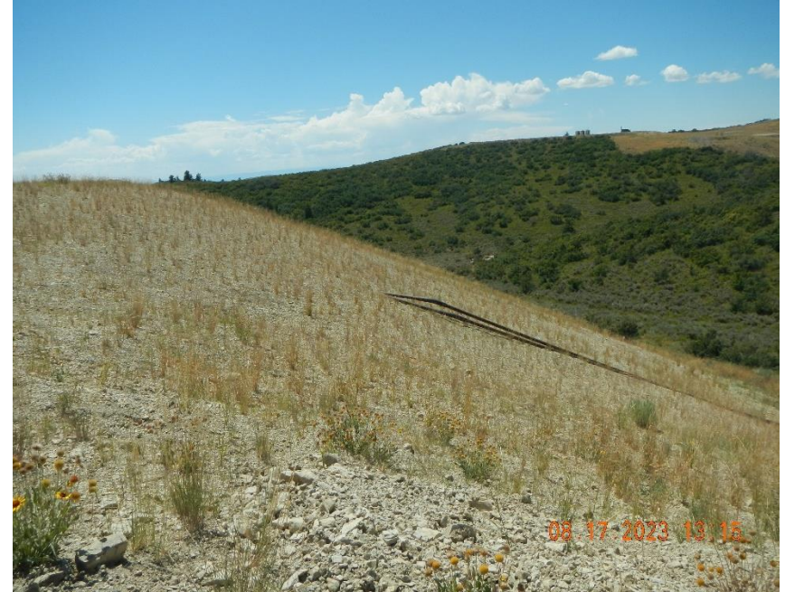
2 – 4" unused flowlines at north west edge of location.
