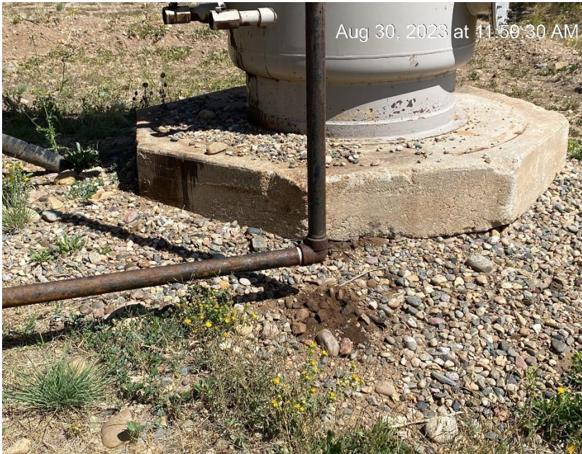
Leak? Stained soil
