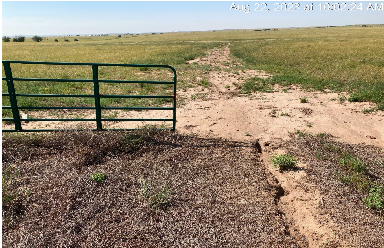
Photo 1. Facing south along the former access road which has not established vegetation. There are some signs of erosion along the road.
