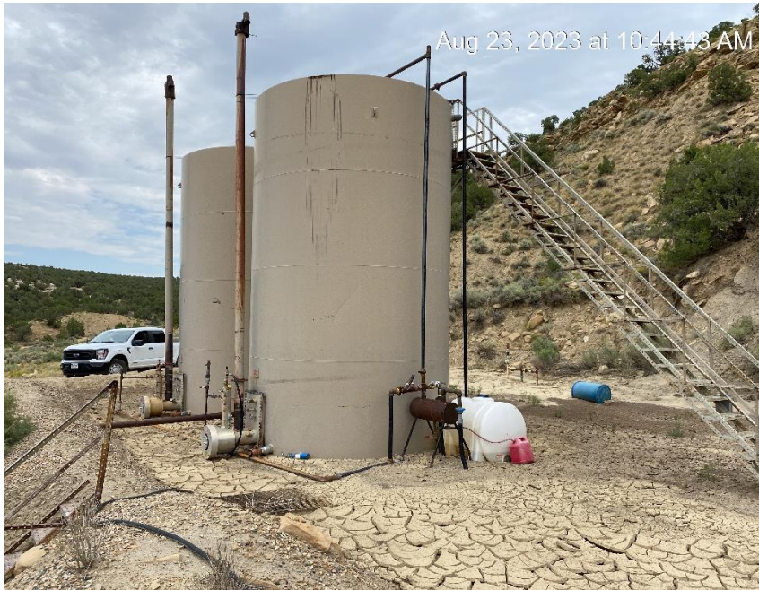
Tank battery. Stormwater BMPs not in place.
