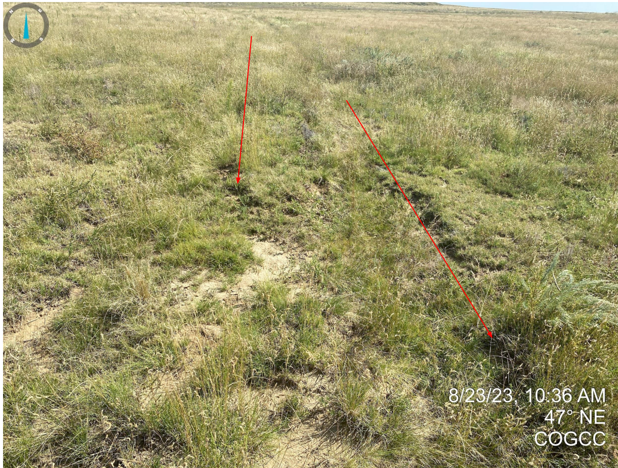
Photo 7. Taken from the north-south access road. Heavy rutting on the former access road (obscured by vegetation) will require additional reclamation activities in order to comply with Rule 1004.
