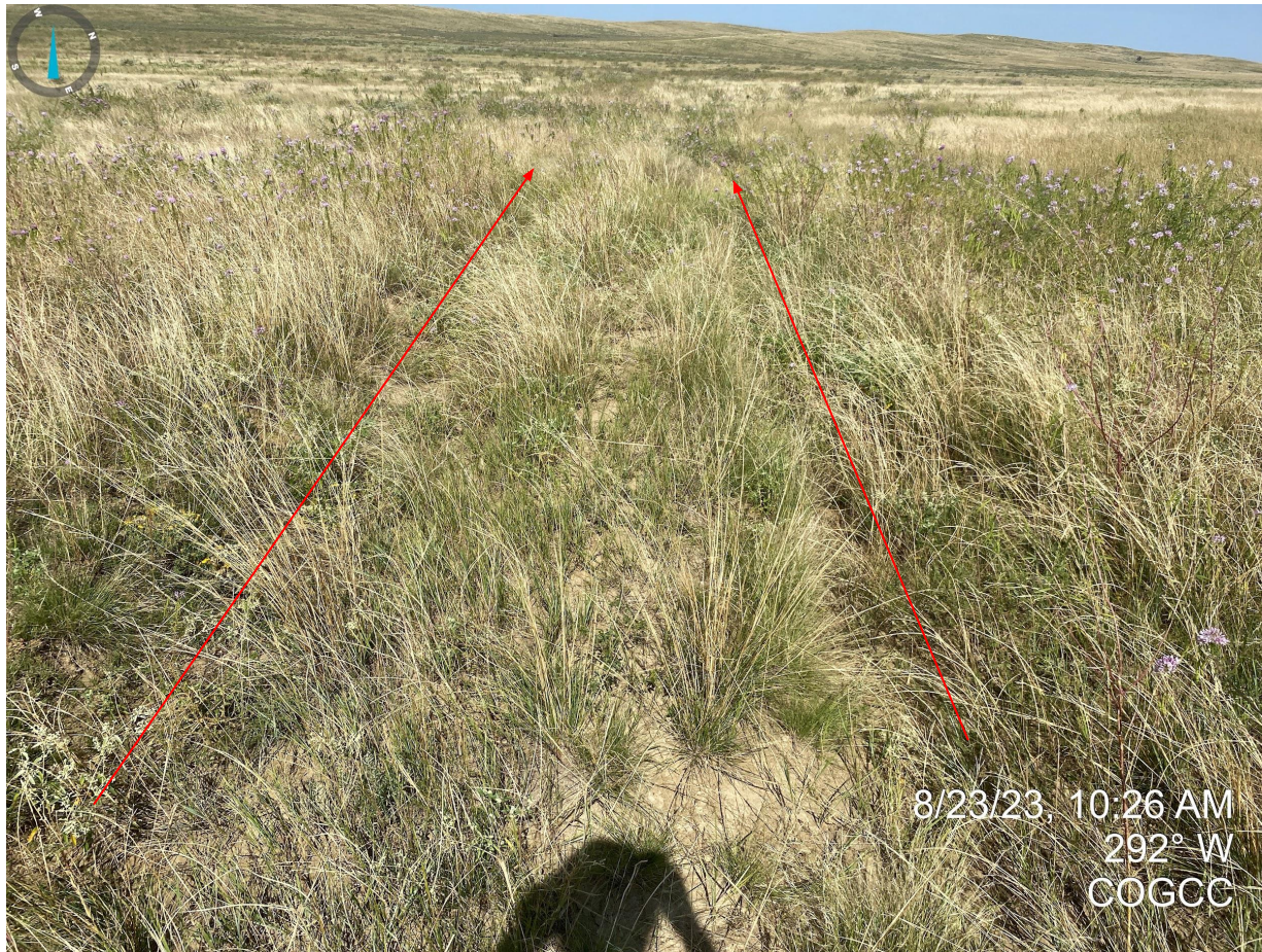
Photo 4. Taken on the east-west lease road. Heavy rutting on the former access road (obscured by vegetation) will require additional reclamation activities in order to comply with Rule 1004.
