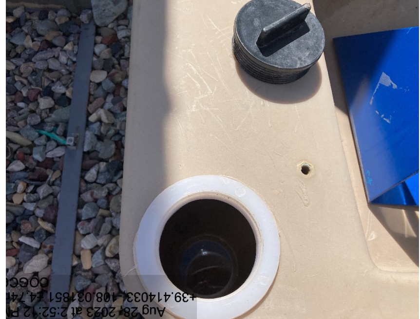
Chemical tank containment is full of fluid
