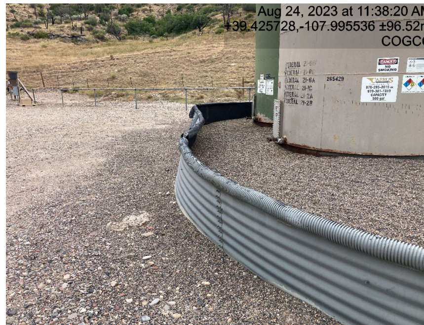
Tank containment has been run into
