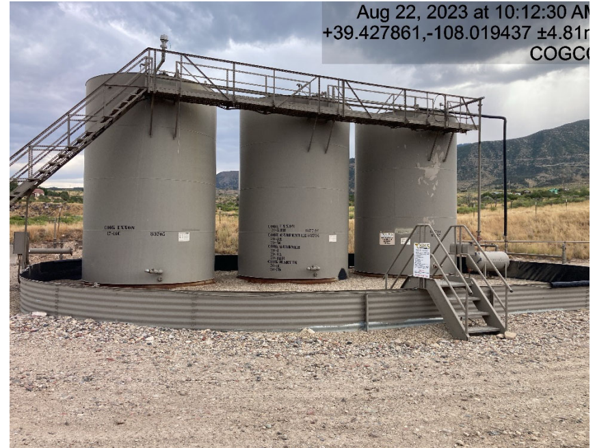
Tank battery lacking proper signage
