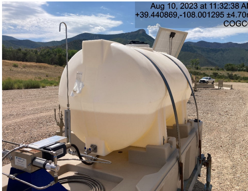
Tank lacking labeling
