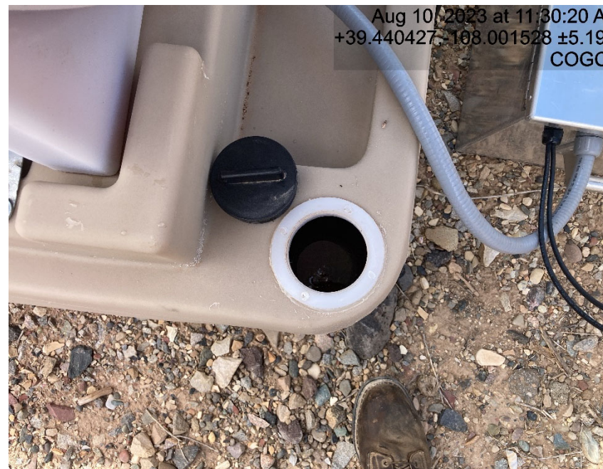
Chemical tank containment is full of fluid
