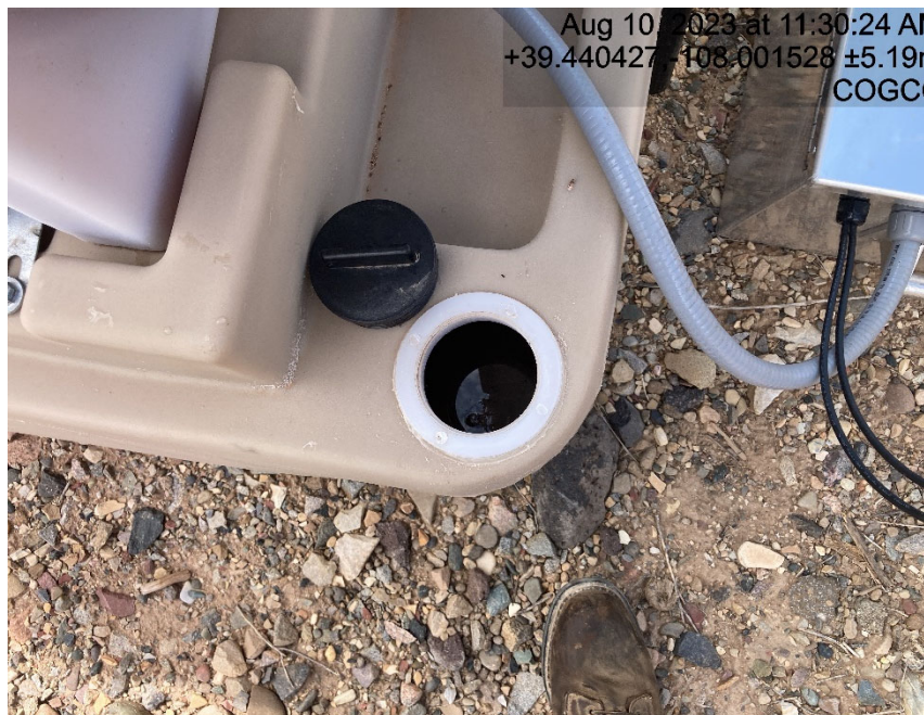
Chemical tank containment is full of fluid
