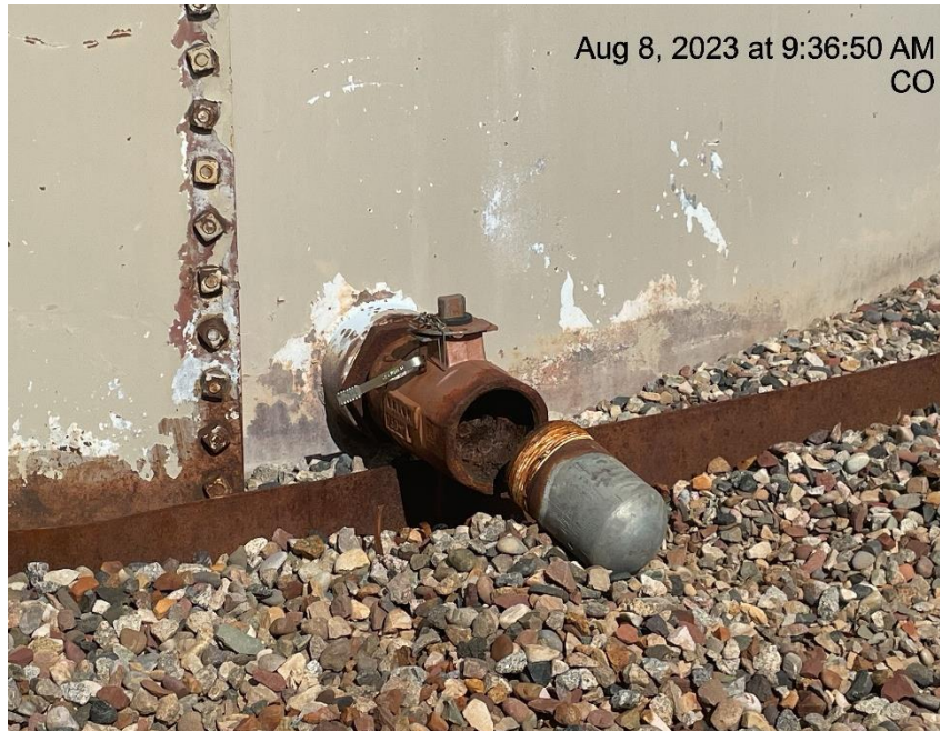
Photo # 5161 From inspection 708901316 conducted on 08/08/2023 Open ended load line
