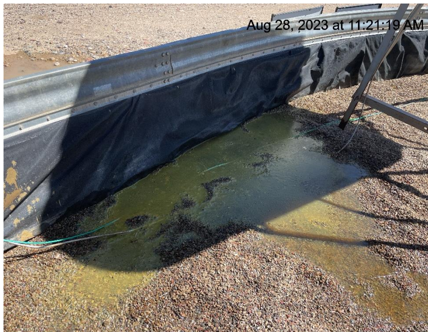
Photo # 7469 E & P waste in secondary containment
