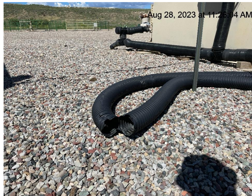
Photo # 7480 Flowline heating insulation open ended
