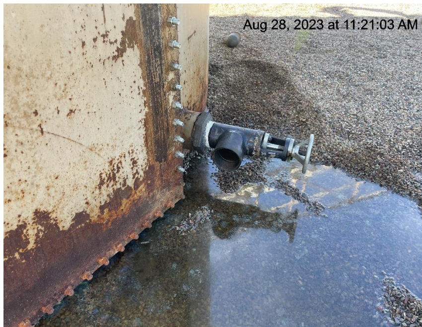
Photo # 7467 Open ended load line/stained gravel
