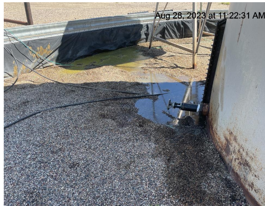
Photo # 7475 E & P waste in secondary containment/stained gravel
