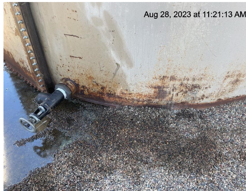
Photo # 7468 Stained gravel in secondary containment
