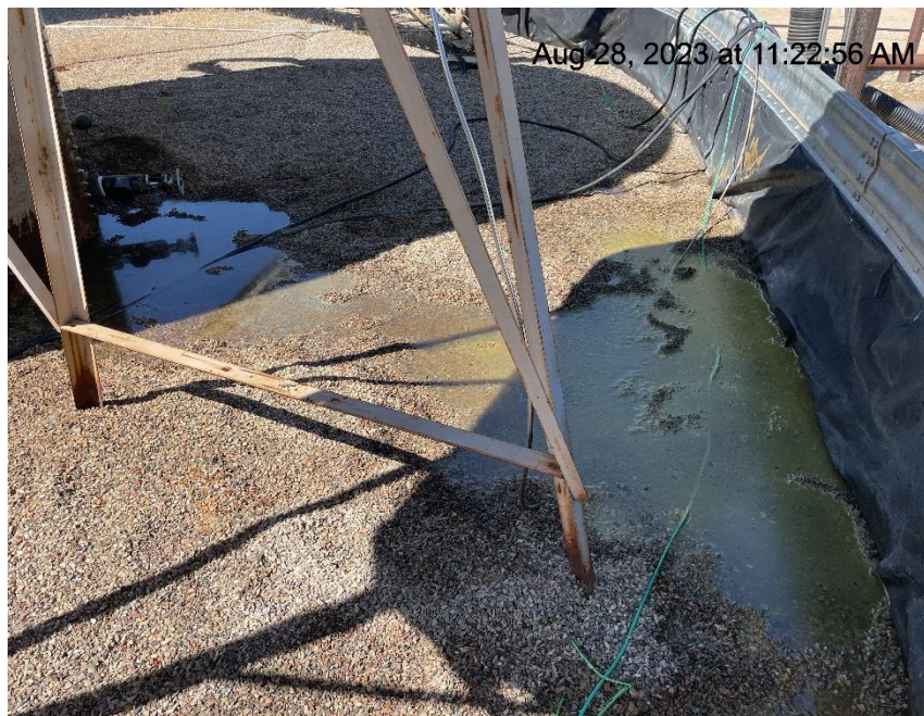
Photo # 7476 E & P waste in secondary containment
