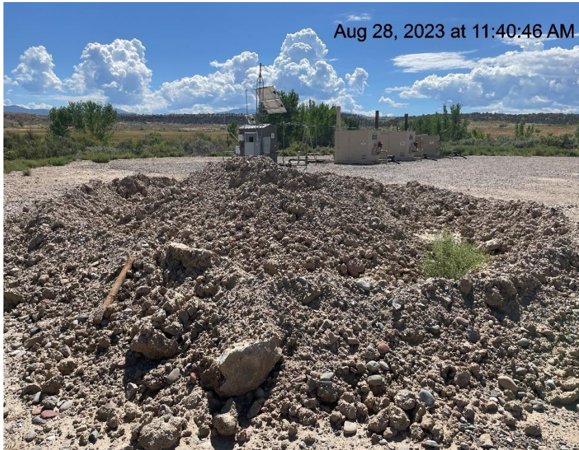
Photo # 7494 Stockpiled soils/insufficient BMP's
