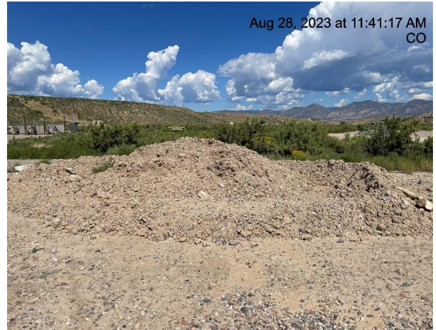
Photo # 7496 Stockpiled soils/insufficient BMP's
