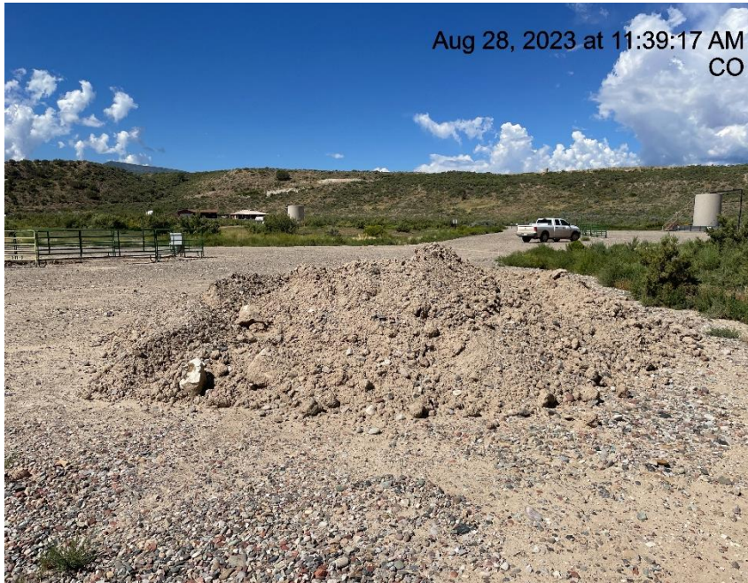
Photo # 7490 Stockpiled soils/insufficient BMP's
