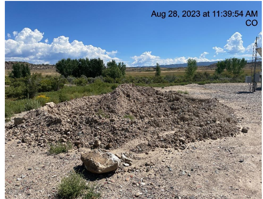
Photo # 7492 Stockpiled soils/insufficient BMP's
