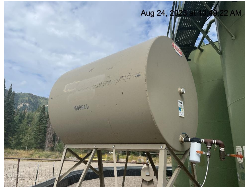
Photo # 7112 Methanol tank lacks required information
