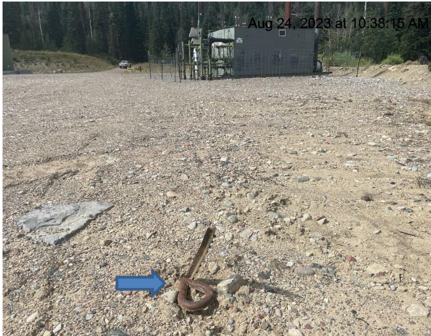
Photo # 7096 Improperly marked deadman
