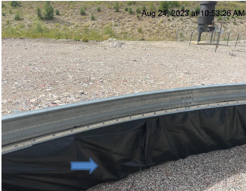
Photo # 7124 Hole in liner/liner needs maintenance
