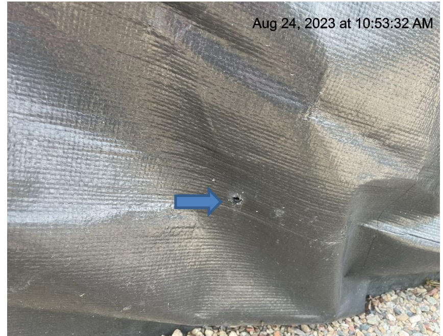
Photo # 7125 Hole in liner/liner needs maintenance
