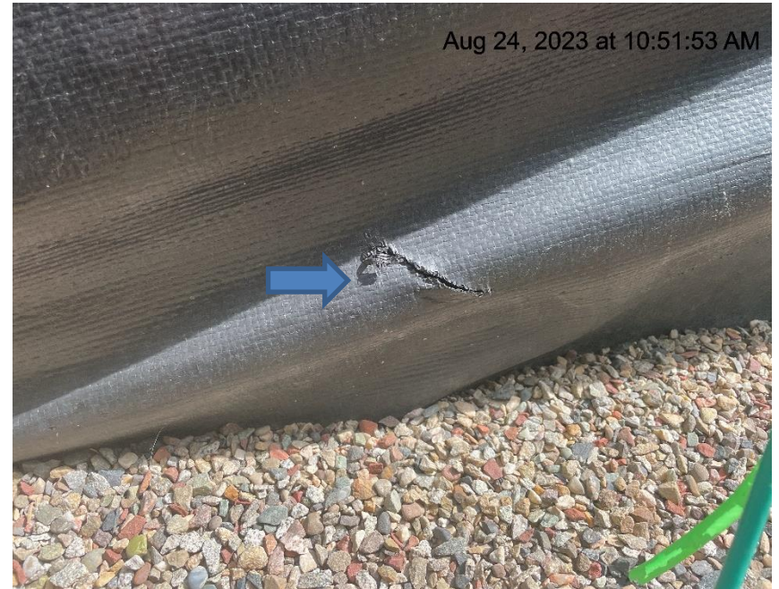
Photo # 7116 Hole in liner/liner needs maintenance
