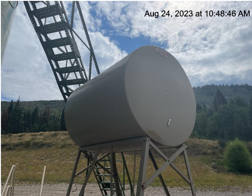
Photo # 7111 Methanol tank lacks required information
