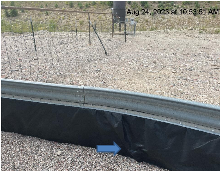
Photo # 7126 Hole in liner/liner needs maintenance
