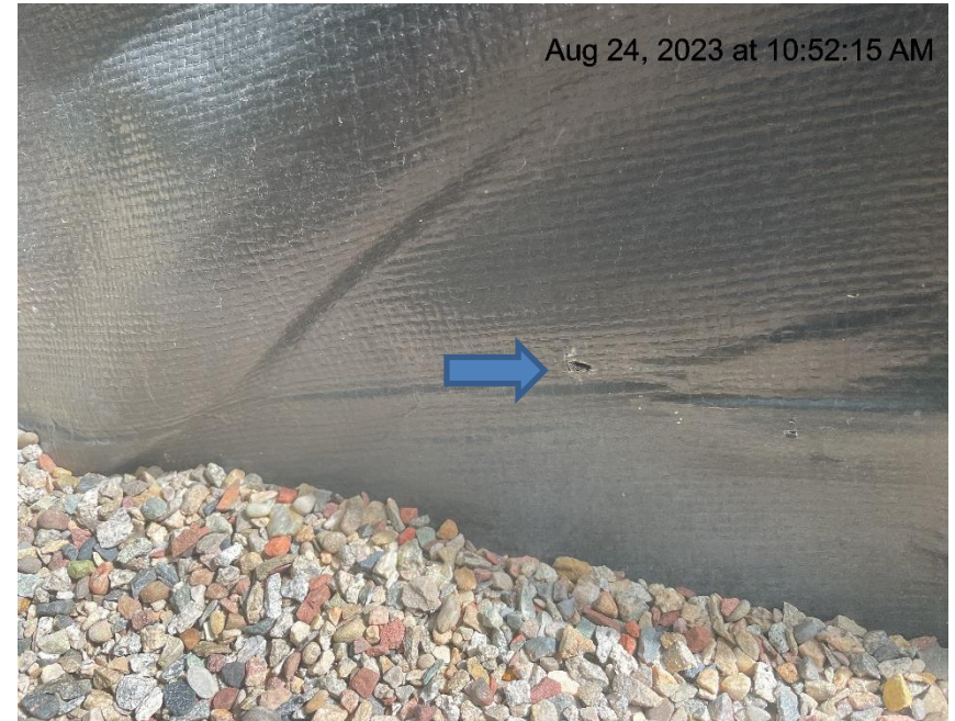
Photo # 7119 Hole in liner/liner needs maintenance
