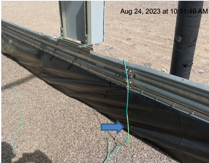
Photo # 7115 Hole in liner/liner needs maintenance
