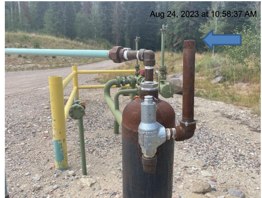
Photo # 7136 PRV vent lacks cap
