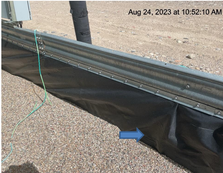
Photo # 7118 Hole in liner/liner needs maintenance
