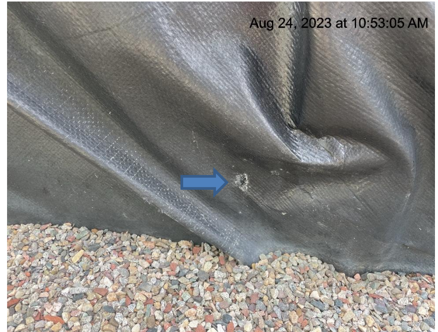
Photo # 7122 Hole in liner/liner needs maintenance
