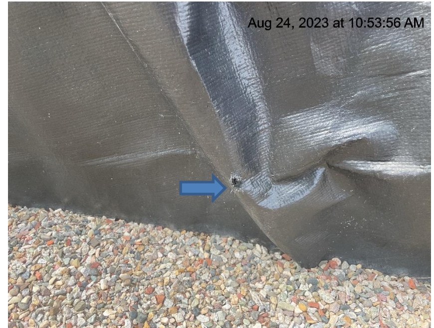
Photo # 7127 Hole in liner/liner needs maintenance
