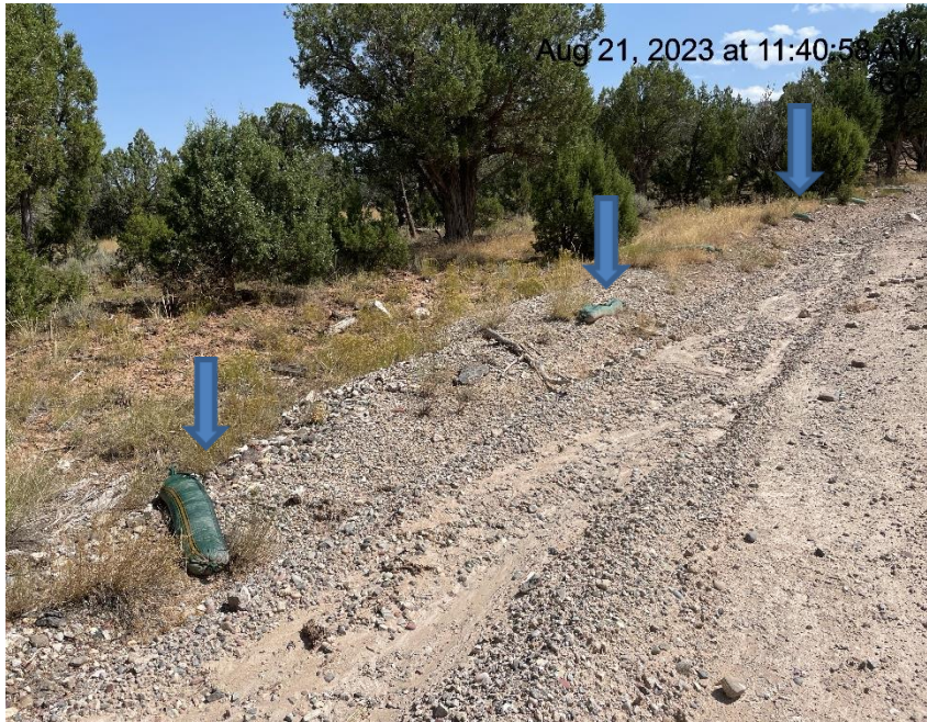
Photo # 6909 Rock socks/BMP's laying along side road & not in use in multiple areas
