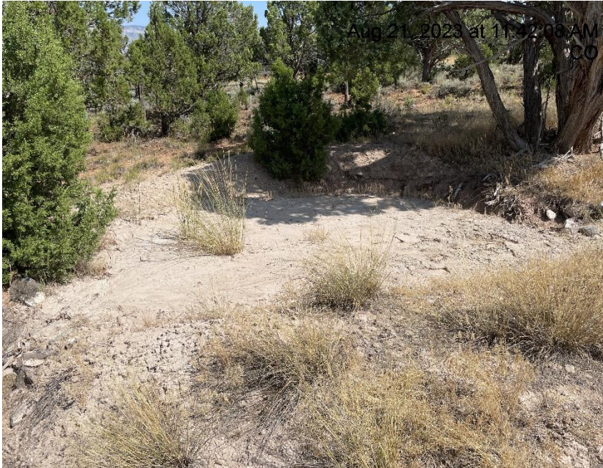
Photo # 6915 Sediment trap needs maintenance (approximately 20-30 yards after you turn onto spur road to location)
