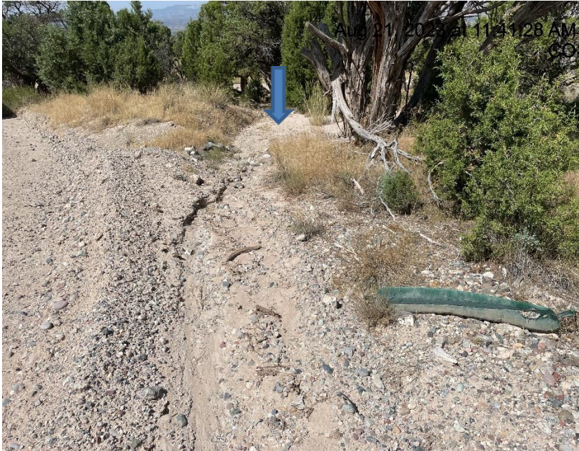
Photo # 6912 Sediment trap needs maintenance (approximately 20-30 yards after you turn onto spur road to location)
