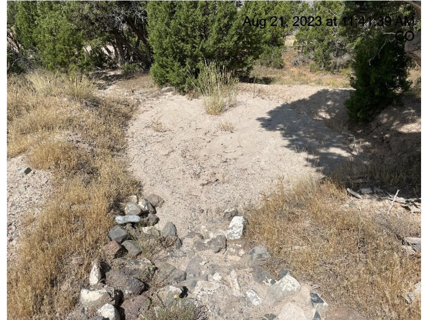
Photo # 6914 Sediment trap needs maintenance (approximately 20-30 yards after you turn onto spur road to location)
