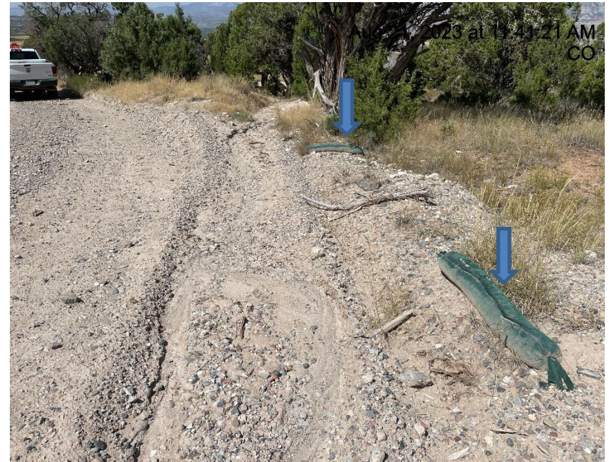
Photo # 6911 Rock socks/BMP's laying along side road & not in use in multiple areas
