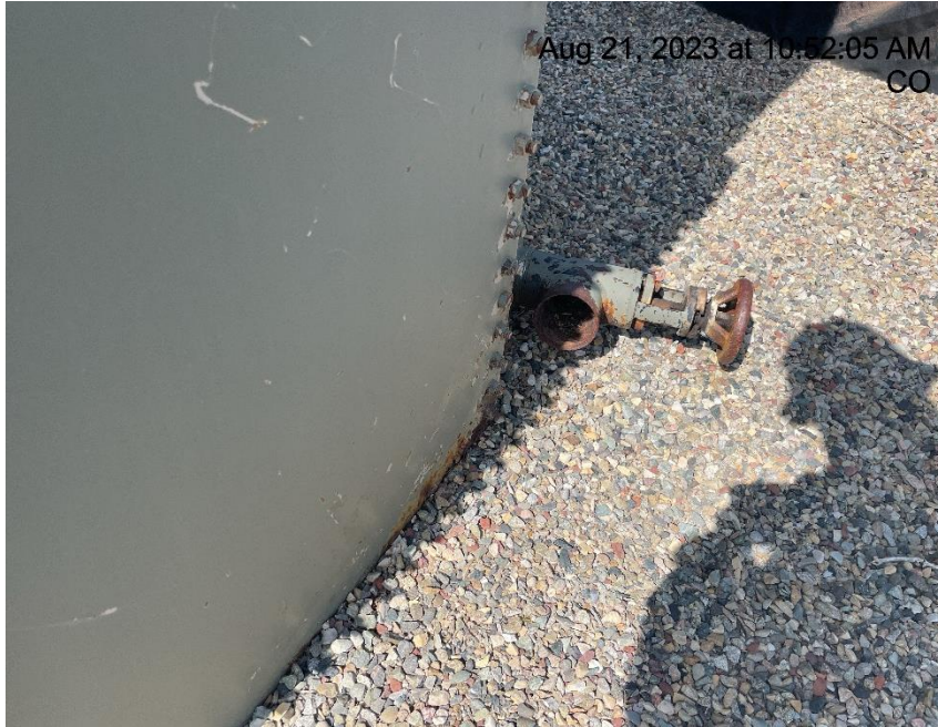
Photo # 6823 Open ended load line
