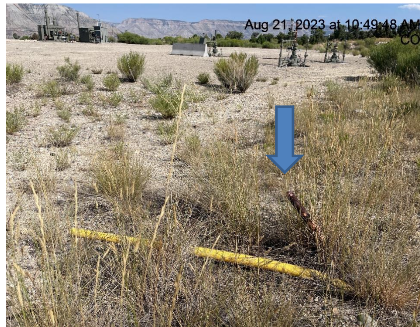
Photo # 6817 Improperly marked deadman
