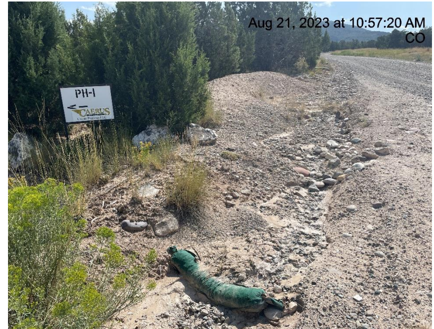
Photo # 6836 Erosion & transport of sediment/insufficient BMP's
