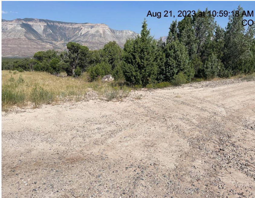
Photo # 6851 Erosion & transport of sediment across road & into a vegetated area/insufficient BMP's
