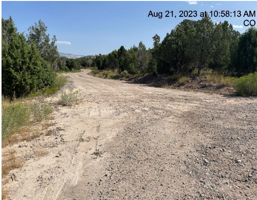
Photo # 6842 Erosion & transport of sediment across road & into a vegetated area/insufficient BMP's
