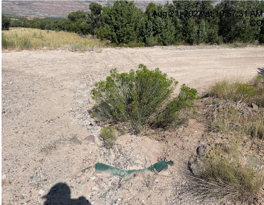
Photo # 6837 Erosion & transport of sediment/insufficient BMP's
