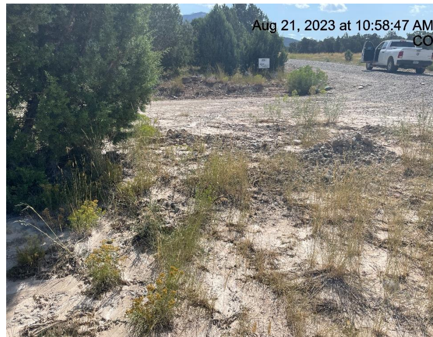
Photo # 6845 Erosion & transport of sediment across road & into a vegetated area/insufficient BMP's
