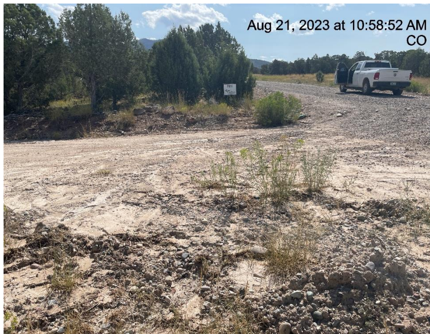
Photo # 6846 Erosion & transport of sediment across road & into a vegetated area/insufficient BMP's
