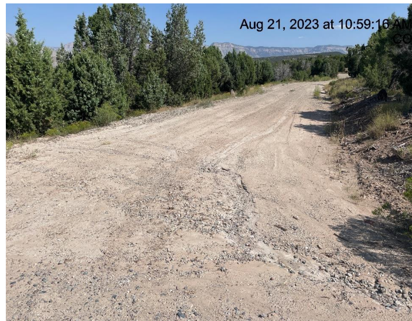
Photo # 6850 Erosion & transport of sediment across road & into a vegetated area/insufficient BMP's
