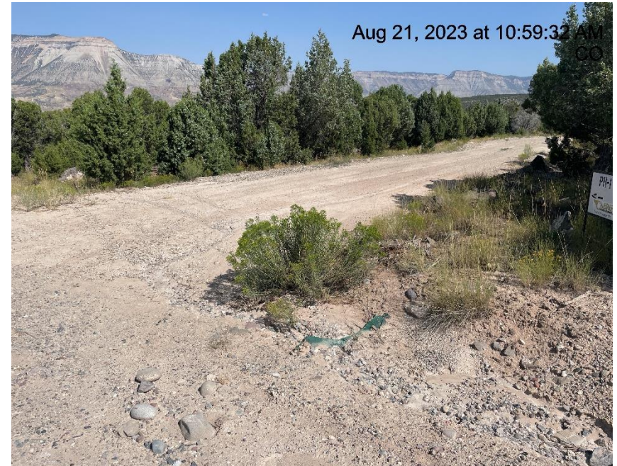
Photo # 6852 Erosion & transport of sediment across road & into a vegetated area/insufficient BMP's
