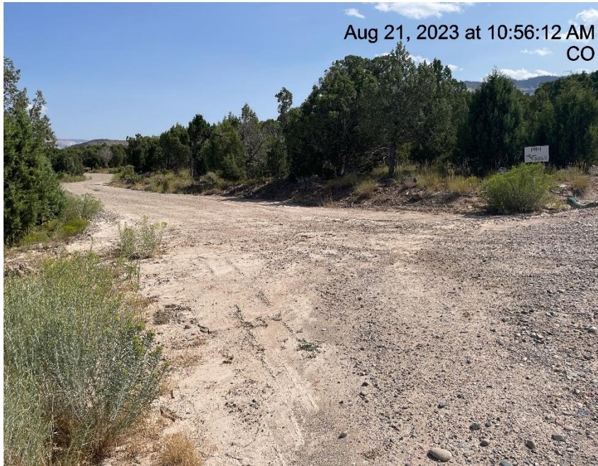
Photo # 6832 Erosion & transport of sediment across spur road to location & into a vegetated area
