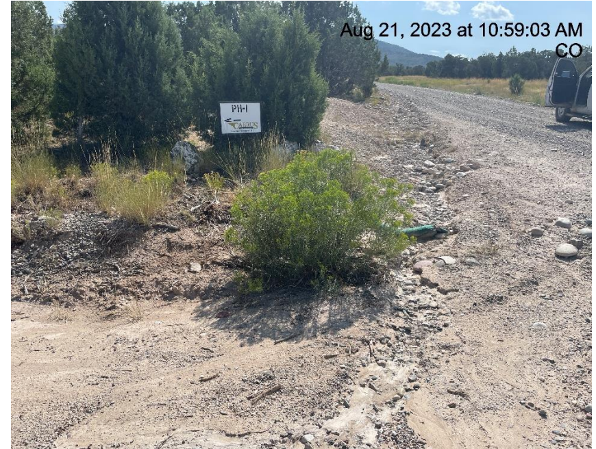
Photo # 6848 Erosion & transport of sediment/insufficient BMP's
