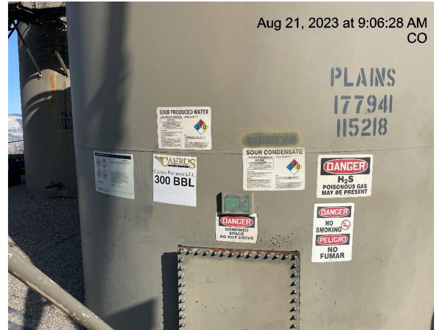
Photo # 6674 Tank/label missing required information
