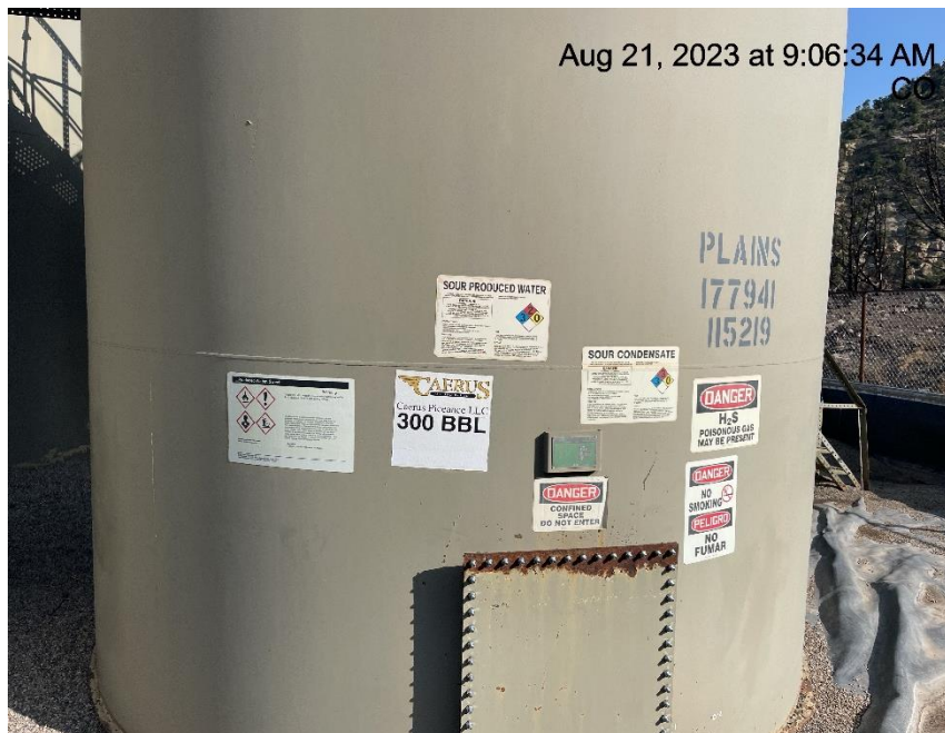
Photo # 6675 Tank/label missing required information
