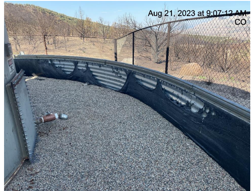
Photo # 6677 Containment liner needs maintenance
