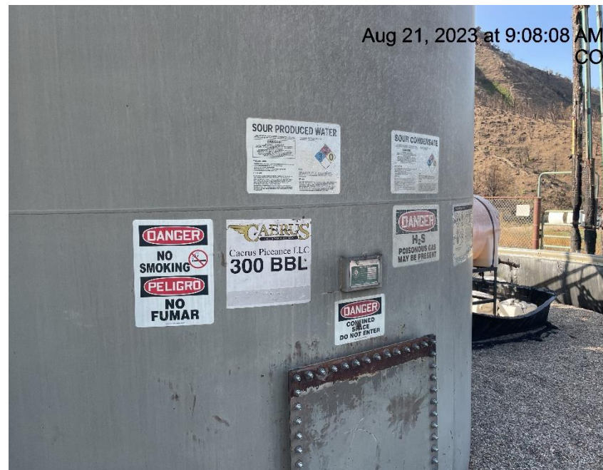
Photo # 6682 Tank/label missing required information
