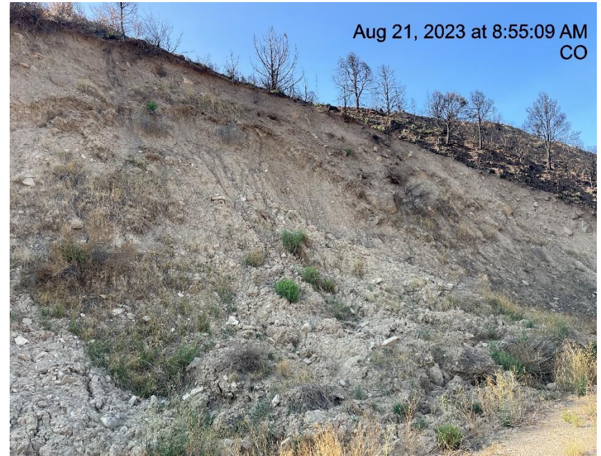
Photo # 6638 Lack of stabilization on cut slope (S/SE area of location)
