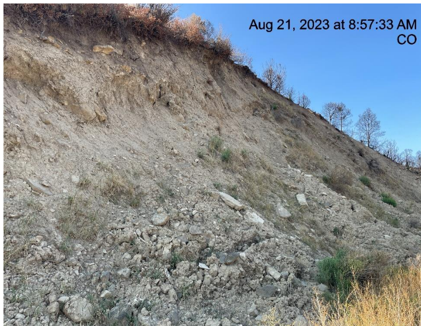
Photo # 6647 Lack of stabilization on cut slope (S/SE area of location)
