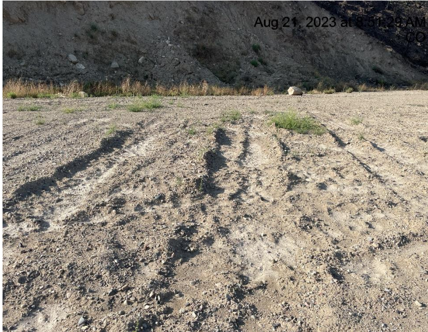
Photo # 6631 Lack of stabilization/compaction
