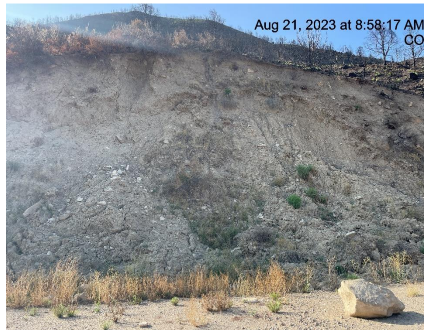
Photo # 6652 Lack of stabilization on cut slope (S/SE area of location)
