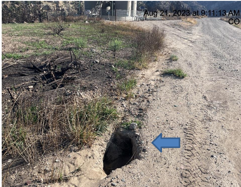
Photo # 6690 Tunnel erosion/sink hole (near entrance to location)
