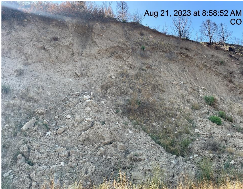
Photo # 6654 Lack of stabilization on cut slope (S/SE area of location)
