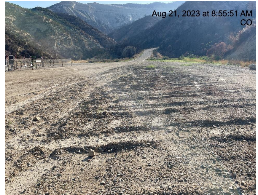
Photo # 6644 Lack of stabilization/compaction
