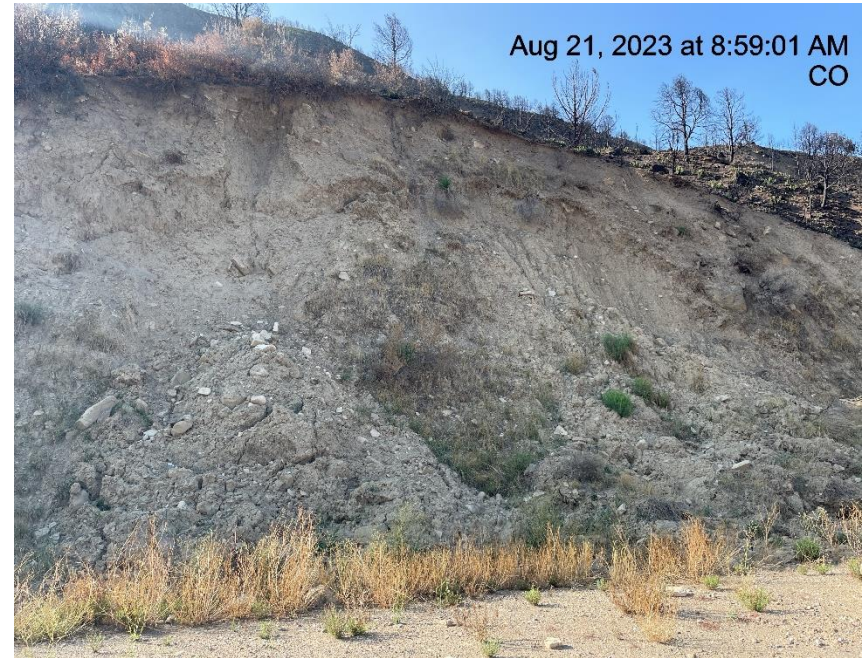
Photo # 6656 Lack of stabilization on cut slope (S/SE area of location)
