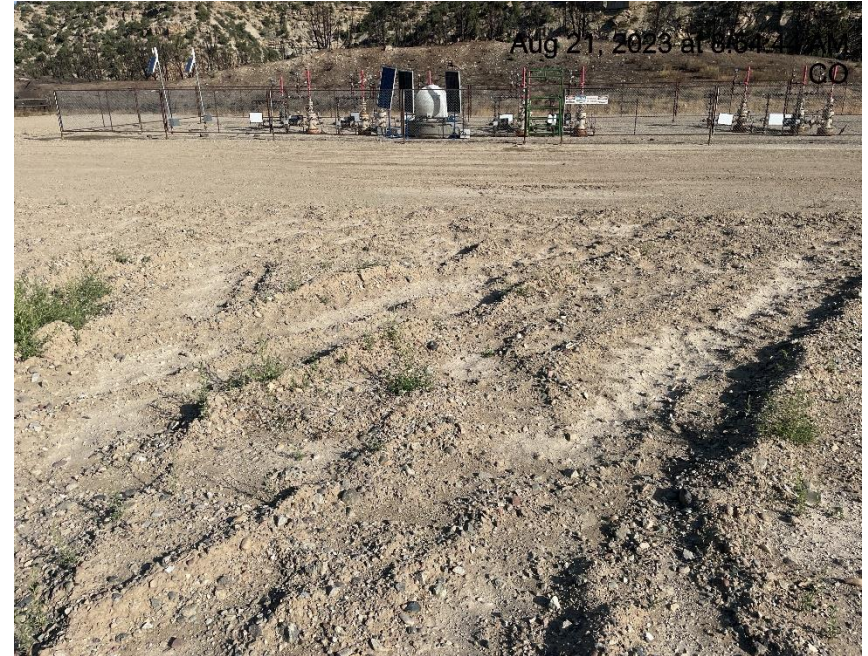
Photo # 6636 Lack of stabilization/compaction
