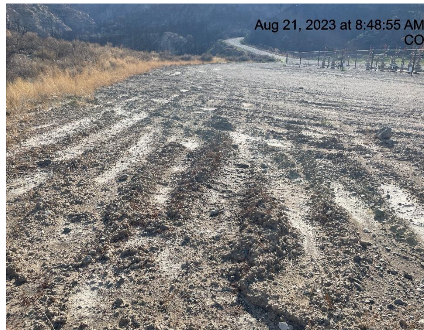
Photo # 6624 Lack of stabilization/compaction
