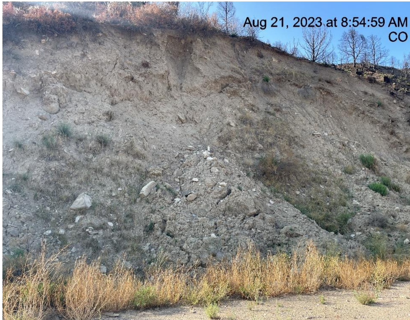
Photo # 6637 Lack of stabilization on cut slope (S/SE area of location)
