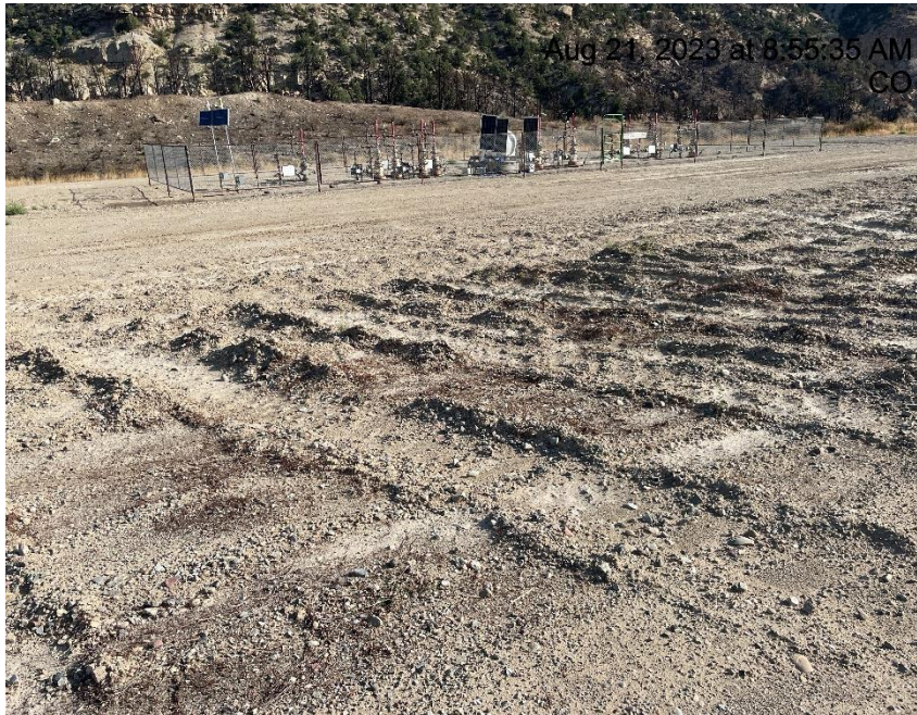
Photo # 6642 Lack of stabilization/compaction
