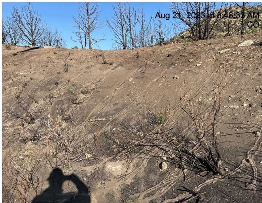
Photo # 6623 Erosion & transport of sediment (N/NE area of location on slope near wellheads)
