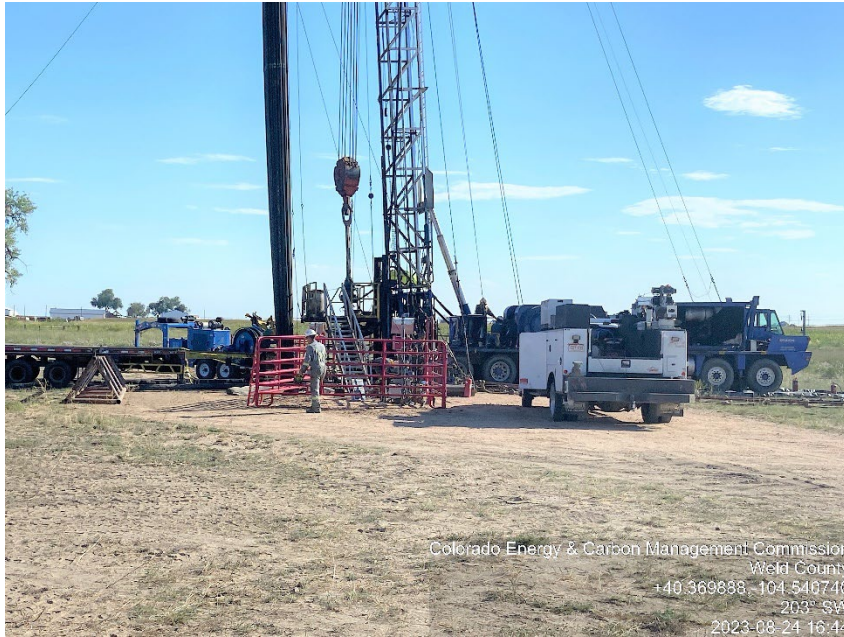
Photo #1 Chesnut 27O-243 (123-39978) Wellsite Workover | WK Workover Ops: Sand clean-out
