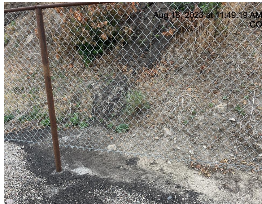
Photo # 6526 Erosion & transport of sediment onto location/insufficient run on controls/BMP's (near tank battery)
