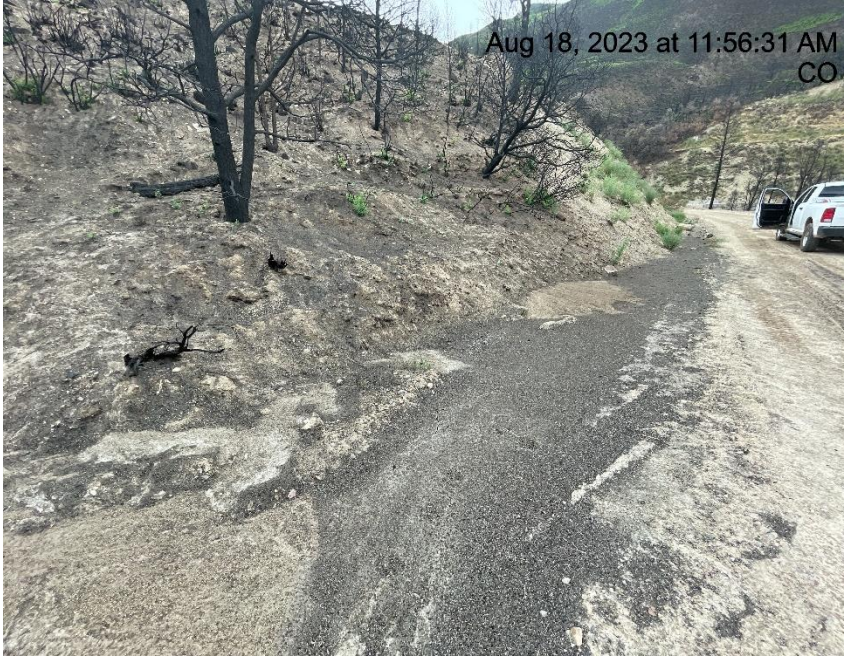
Photo # 6545 Lack of stabilization on slope/erosion & transport of sediment/insufficient run on controls/BMP's (on lease road near pig station)
