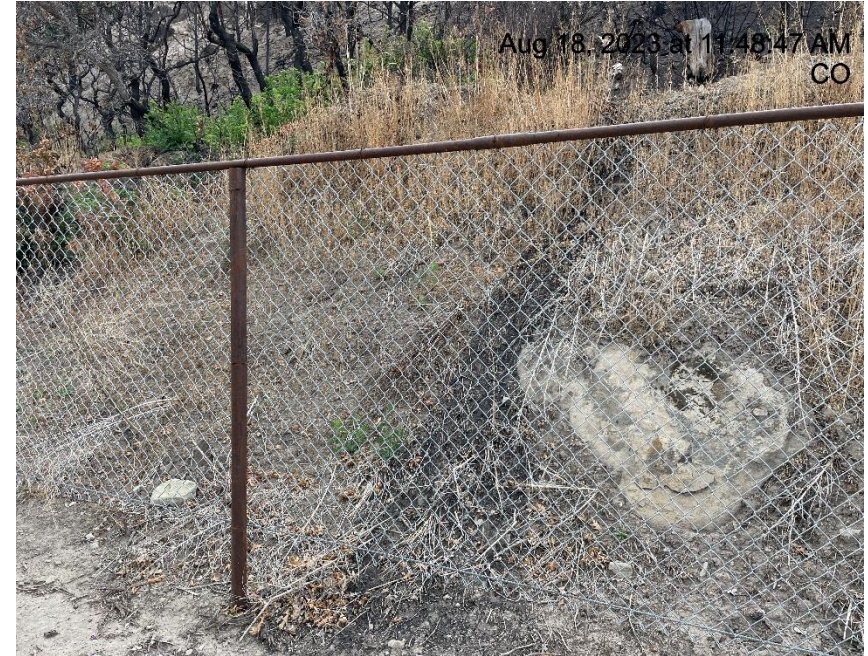
Photo # 6524 Erosion & transport of sediment onto location/insufficient run on controls/BMP's (near tank battery)
