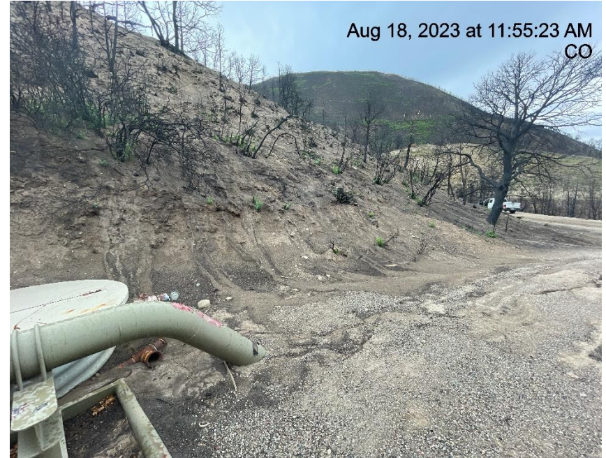
Photo # 6539 Lack of stabilization on slope/erosion & transport of sediment/insufficient run on controls/BMP's
