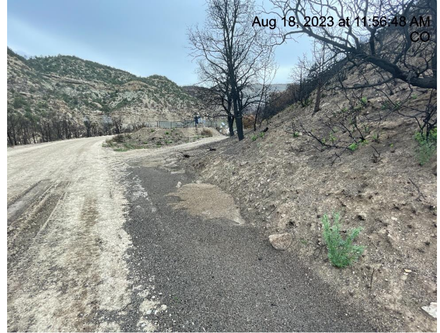
Photo # 6546 Lack of stabilization on slope/erosion & transport of sediment/insufficient run on controls/BMP's (on lease road near pig station)
