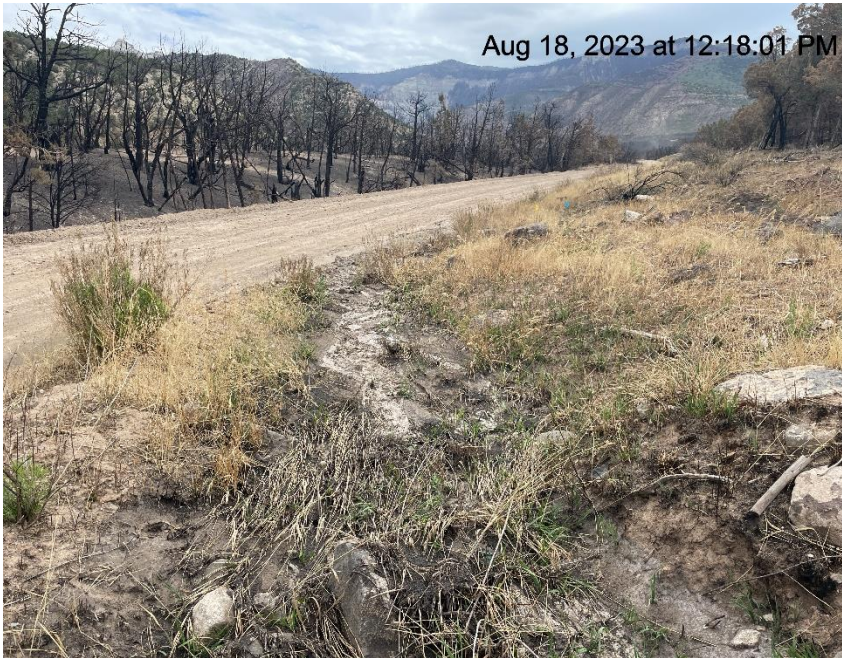
Photo # 6577 Erosion & transport of sediment/BMP's need maintenance (approximately 2 miles from location)
