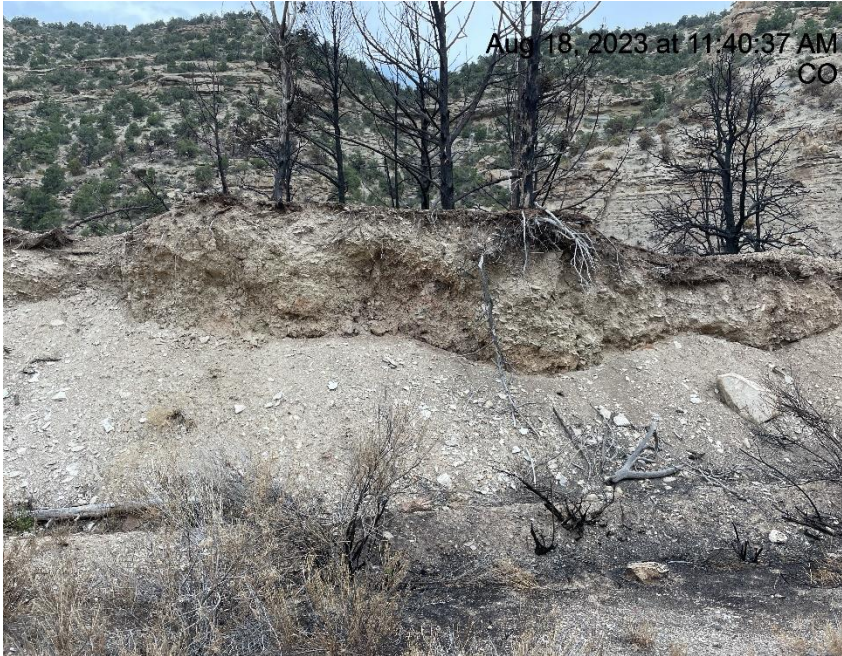
Photo # 6510 Lack of stabilization on slope/insufficient BMP's
