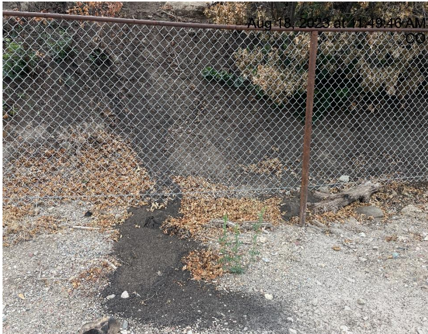
Photo # 6527 Erosion & transport of sediment onto location/lack of stabilization on slope/insufficient run on controls/BMP's (near tank battery)
