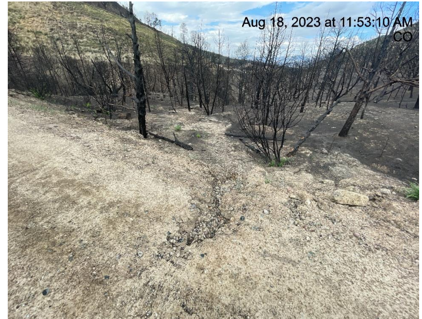
Photo # 6533 Erosion & transport of sediment off lease road (on lease road near pig station)
