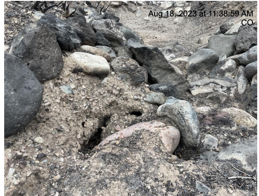
Photo # 6509 BMP needs maintenance, erosion starting to undercut armoring
