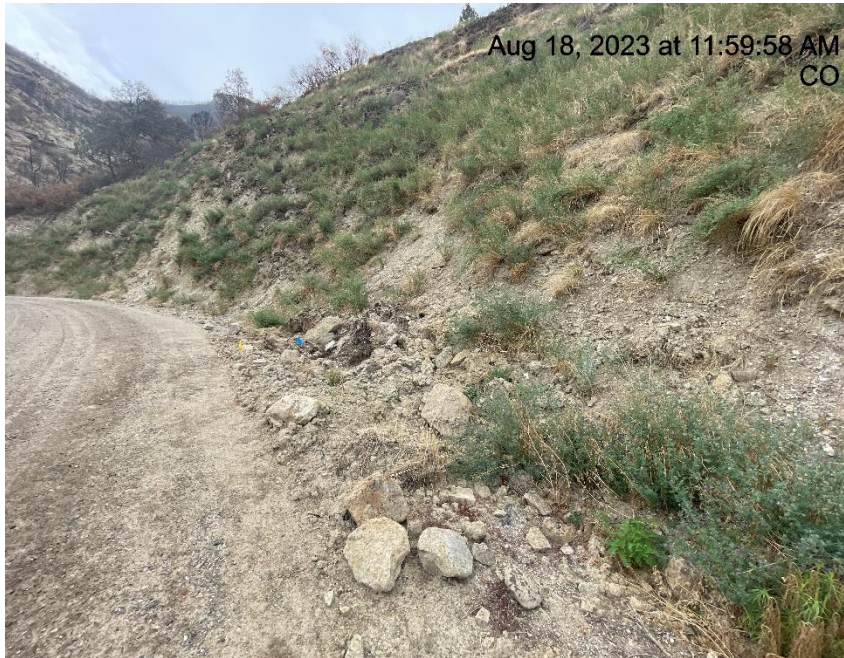
Photo # 6557 Lack of stabilization on slope/transport of sediment onto edge of lease road (approximately 1/10 th of a mile from location)
