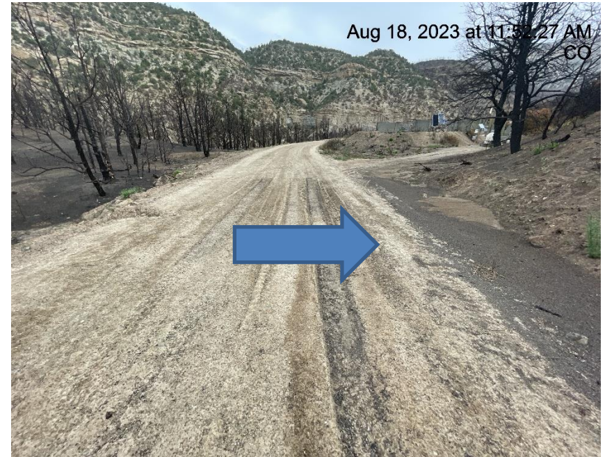
Photo # 6531 Lack of stabilization on slope/erosion & transport of sediment/ditch needs maintenance
