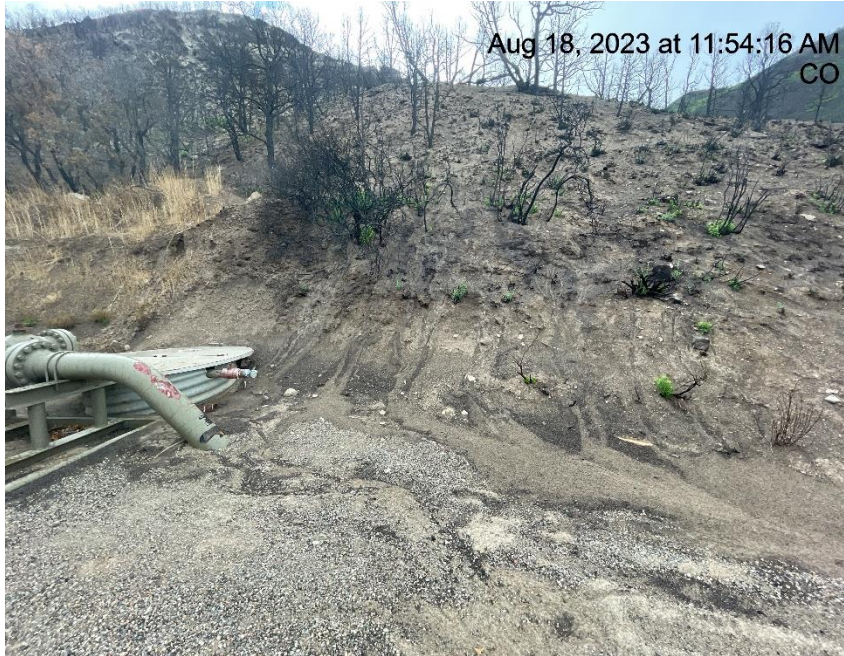
Photo # 6535 Lack of stabilization on slope/erosion & transport of sediment/insufficient run on controls/BMP's
