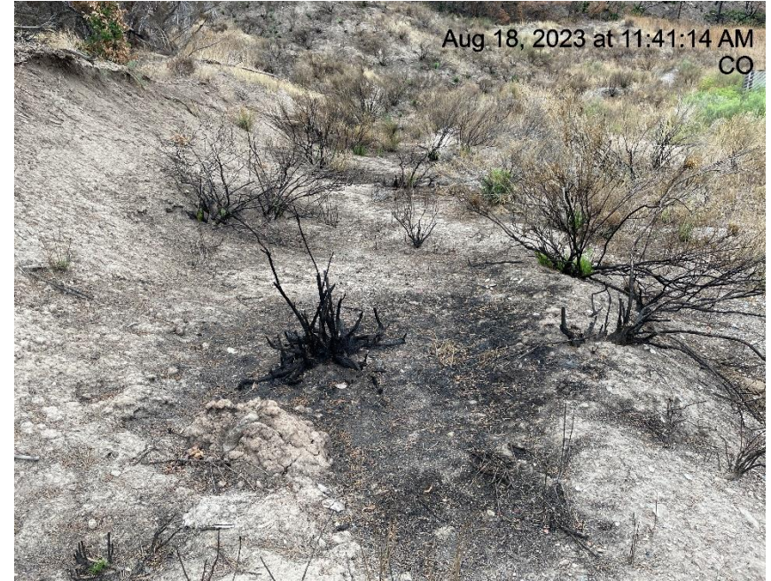
Photo # 6511 Lack of stabilization on slope/insufficient BMP's/ditch needs maintenance
