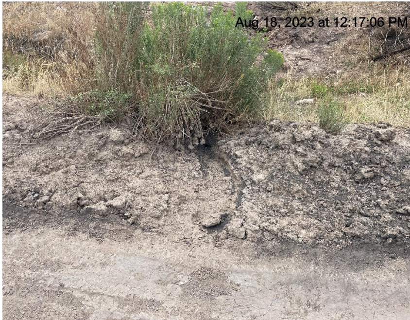
Photo # 6573 Erosion & transport of sediment off lease road (approximately 2 miles from location)
