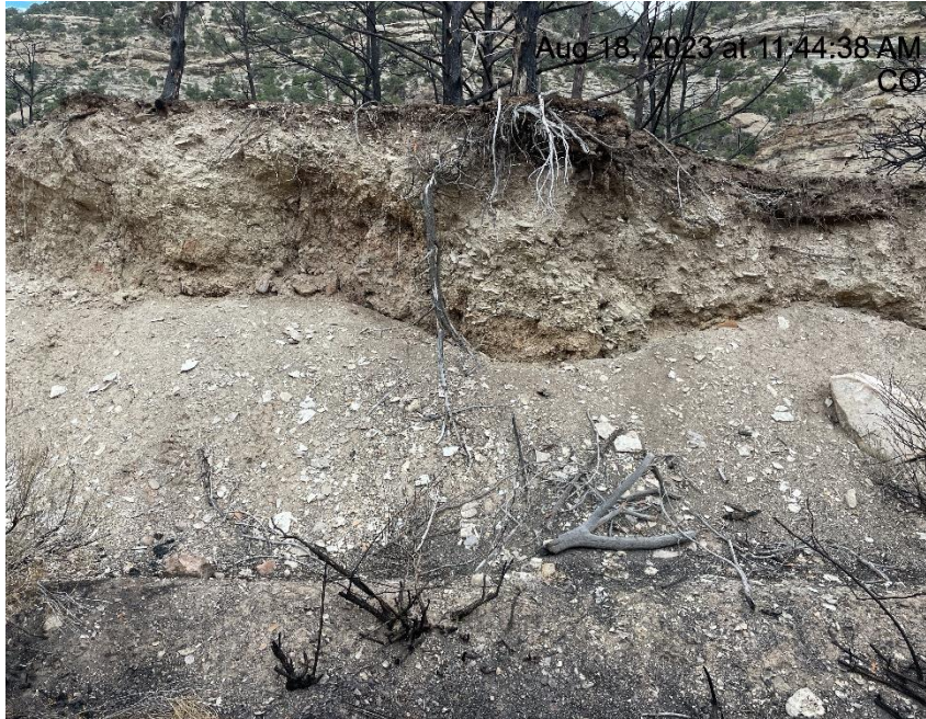
Photo # 6515 Lack of stabilization on slope/insufficient BMP's
