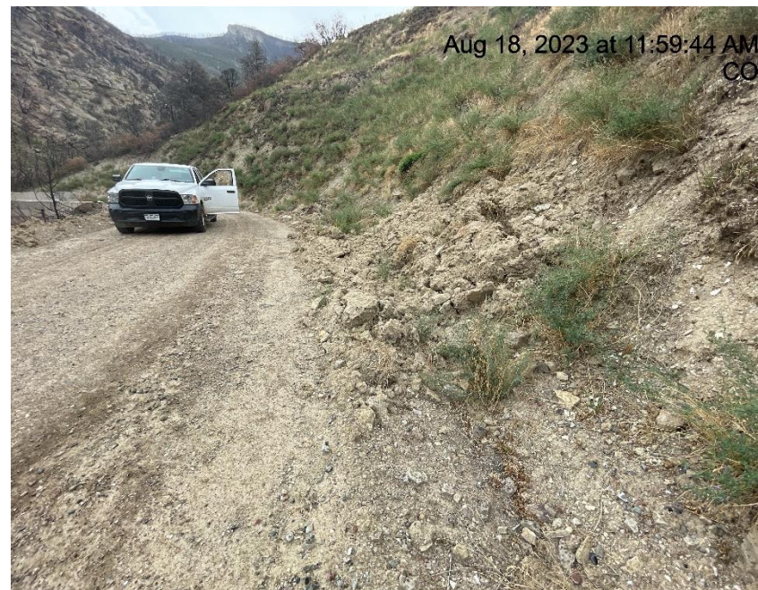
Photo # 6556 Lack of stabilization on slope/transport of sediment onto edge of lease road (approximately 1/10 th of a mile from location)
