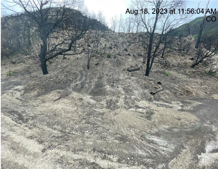
Photo # 6542 Lack of stabilization on slope/erosion & transport of sediment/insufficient run on controls/BMP's (on lease road near pig station)
