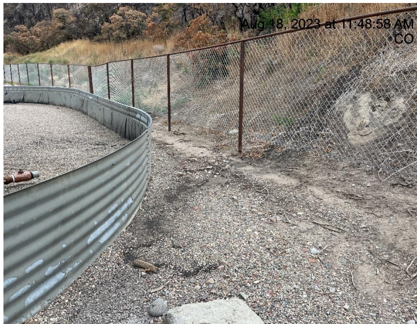
Photo # 6525 Erosion & transport of sediment onto location/insufficient run on controls/BMP's (near tank battery)
