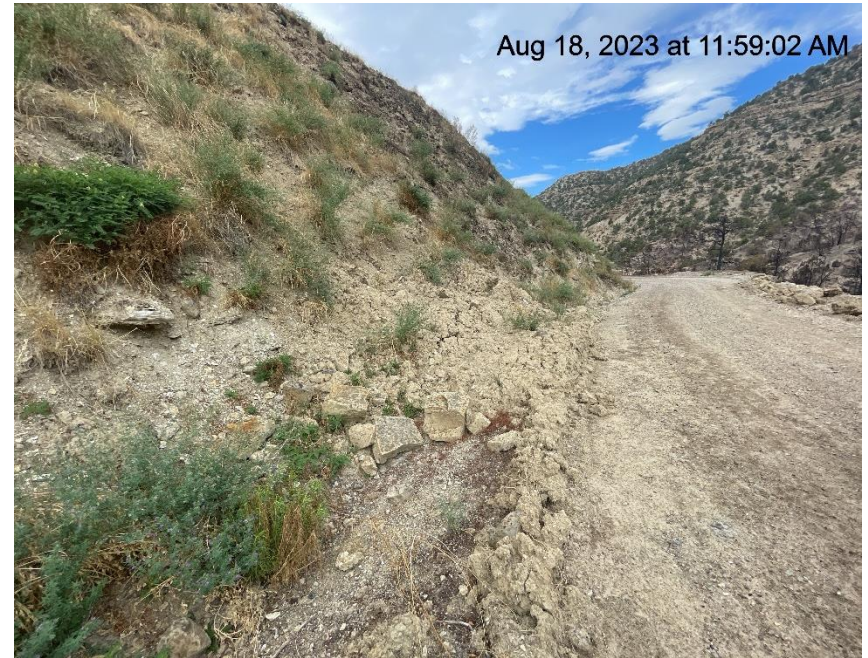
Photo # 6552 Lack of stabilization on slope/transport of sediment onto edge of lease road (approximately 1/10 th of a mile from location)
