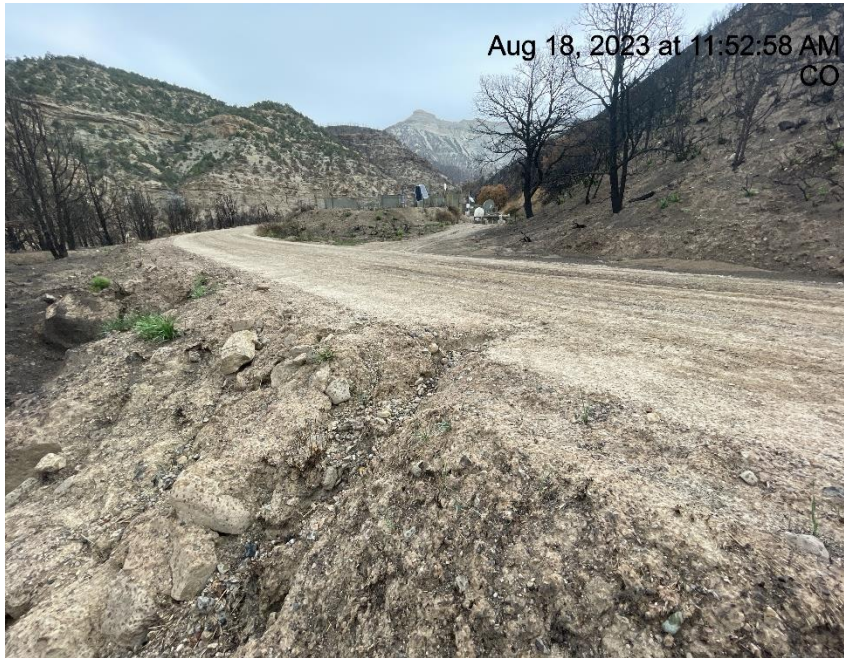
Photo # 6532 Erosion & transport of sediment off lease road (on lease road near pig station)
