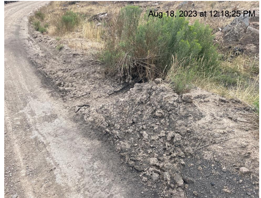
Photo # 6578 Erosion & transport of sediment off lease road (approximately 2 miles from location)
