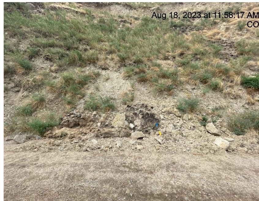
Photo # 6549 Lack of stabilization on slope/transport of sediment onto edge of lease road (approximately 1/10 th of a mile from location)
