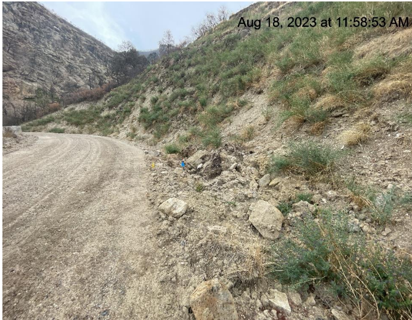
Photo # 6551 Lack of stabilization on slope/transport of sediment onto edge of lease road (approximately 1/10 th of a mile from location)
