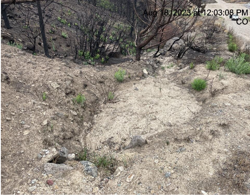
Photo # 6562 Sediment trap needs maintenance (on lease road just after the Federal 8D pad location # 415673)
