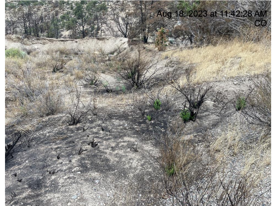
Photo # 6513 Lack of stabilization on slope/insufficient BMP's/ditch needs maintenance
