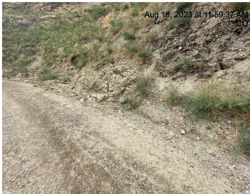
Photo # 6555 Lack of stabilization on slope/transport of sediment onto edge of lease road (approximately 1/10 th of a mile from location)
