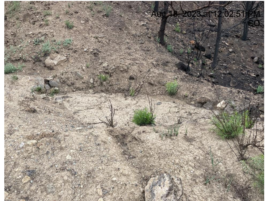
Photo # 6561 Sediment trap needs maintenance (on lease road just after the Federal 8D pad location # 415673)
