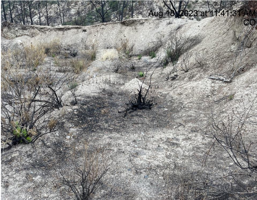
Photo # 6512 Lack of stabilization on slope/insufficient BMP's/ditch needs maintenance
