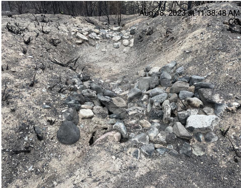
Photo # 6508 BMP needs maintenance, erosion starting to undercut armoring
