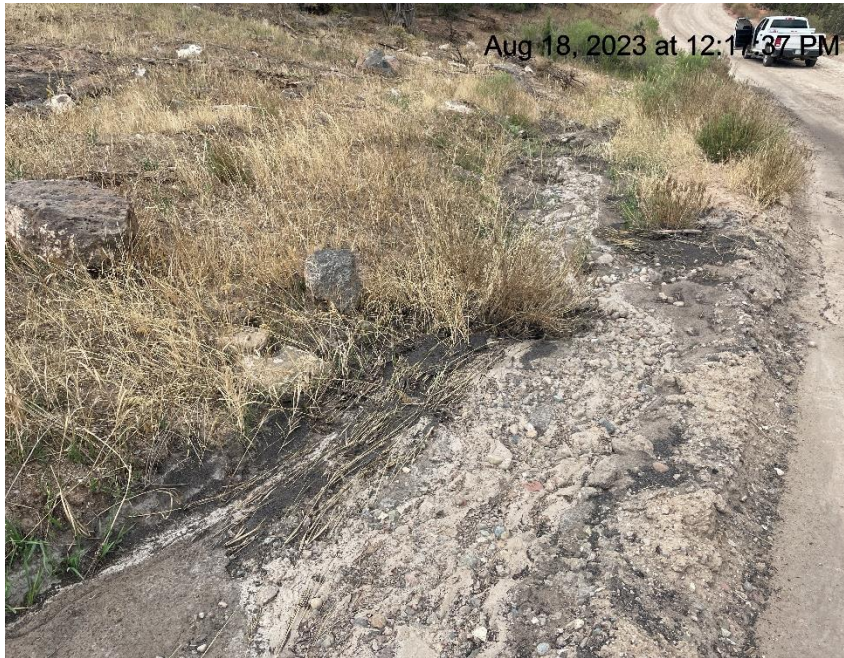
Photo # 6575 Erosion & transport of sediment/BMP's need maintenance (approximately 2 miles from location)
