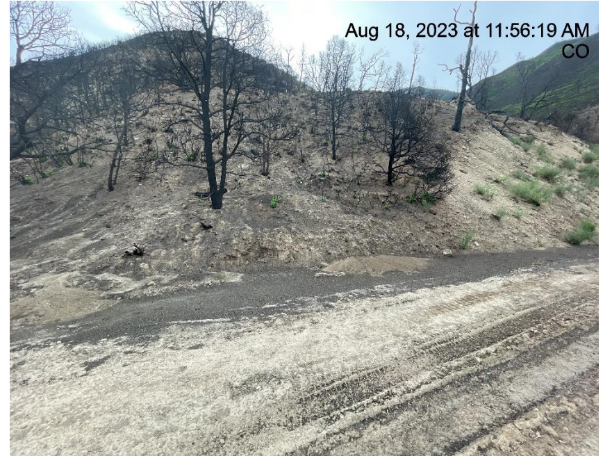
Photo # 6544 Lack of stabilization on slope/erosion & transport of sediment/insufficient run on controls/BMP's (on lease road near pig station)
