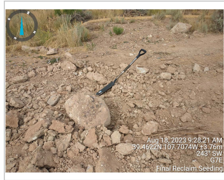
Example of Boulders Surfaced on Road When Using 18" Shanks
