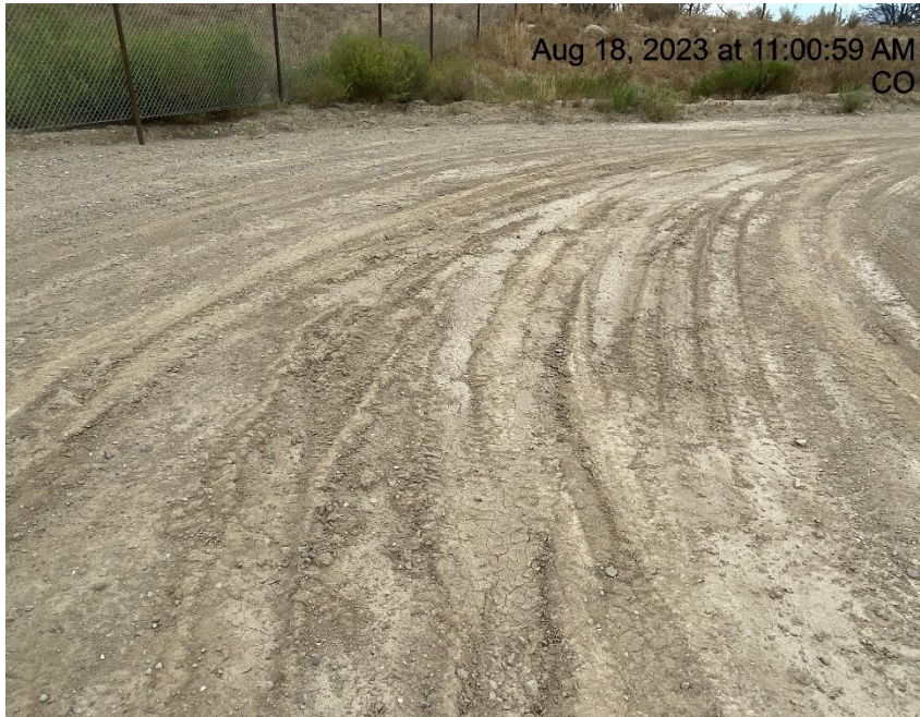
Photo # 6435 Lack of stabilization/compaction
