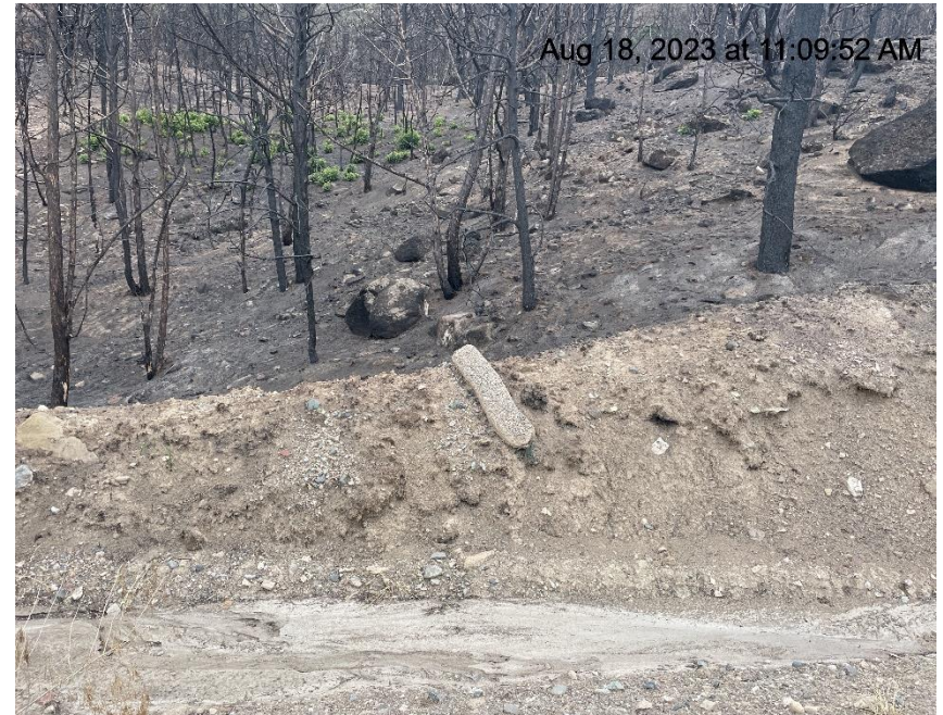
Photo # 6440 Ditch on spur road & BMP's need maintenance
