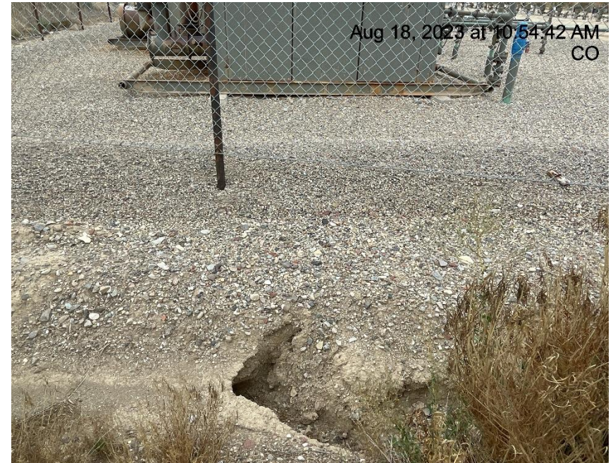
Photo # 6420 Erosion/tunnel erosion (NE corner of location)
