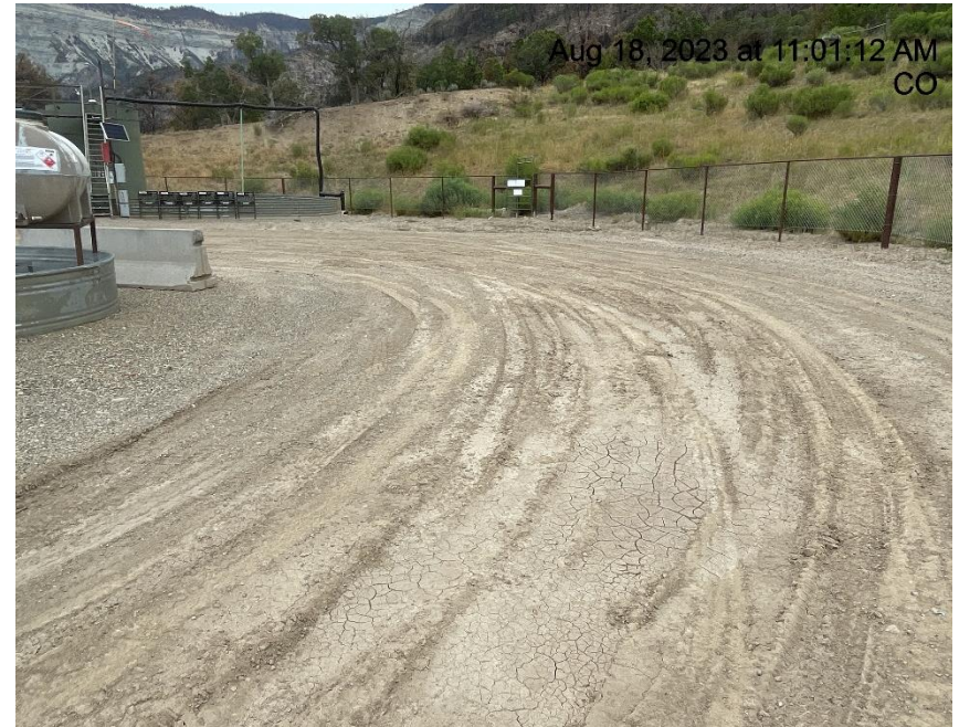
Photo # 6436 Lack of stabilization/compaction
