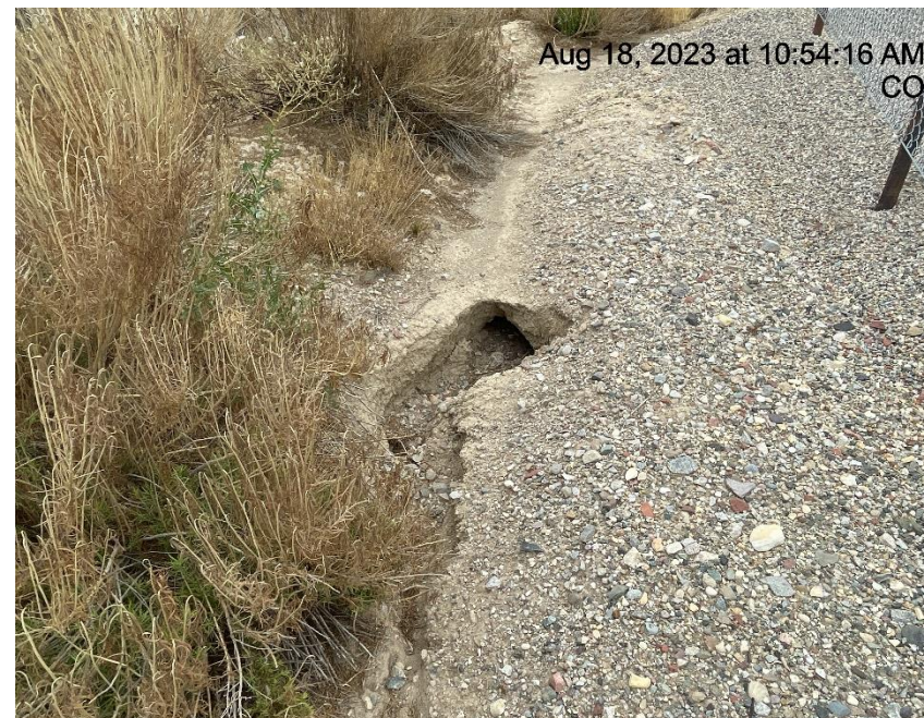
Photo # 6418 Erosion/tunnel erosion (NE corner of location)
