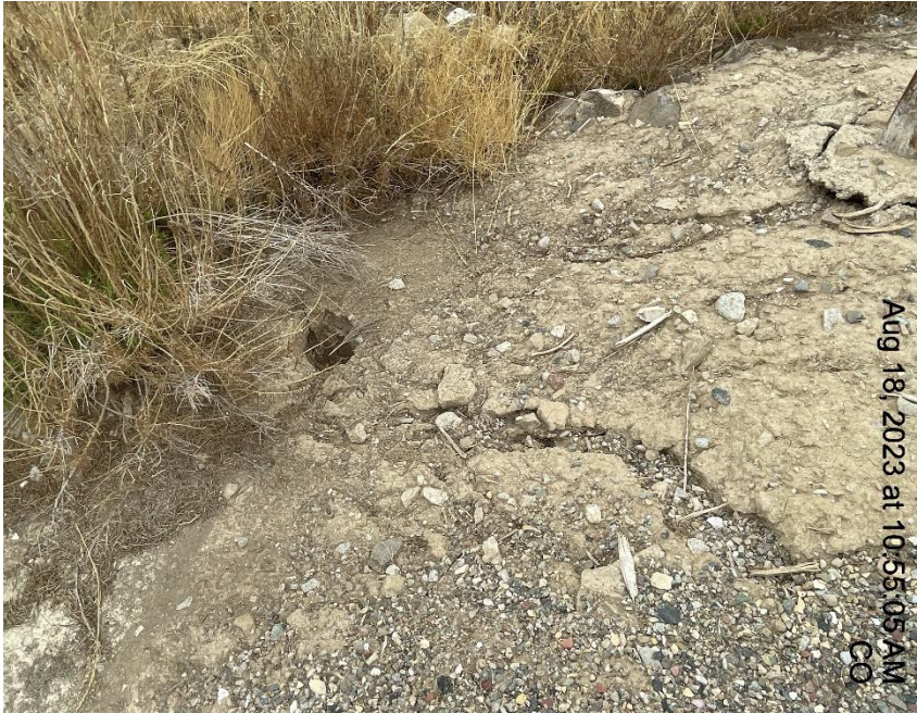
Photo # 6422 Erosion/tunnel erosion (NE corner of location)
