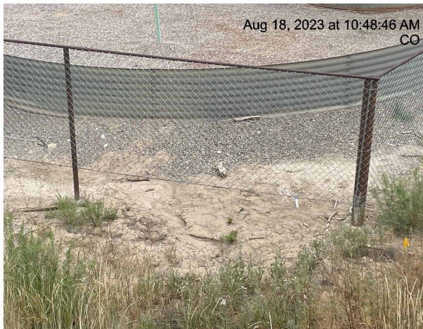
Photo # 6404 Erosion & transport of sediment onto location (SW corner of location)
