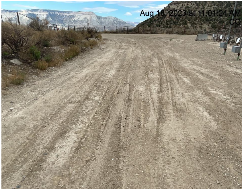
Photo # 6437 Lack of stabilization/compaction
