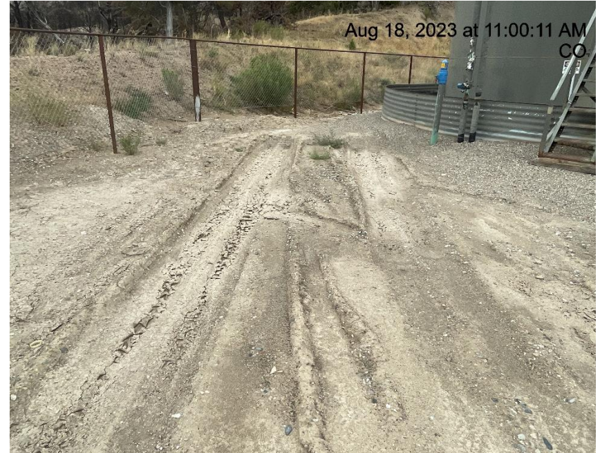
Photo # 6431 Lack of stabilization/compaction
