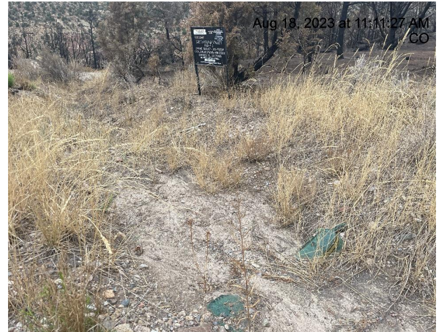
Photo # 6448 Ditch on spur road & check dams need maintenance
