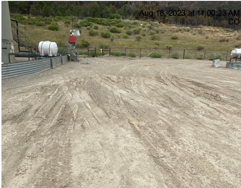
Photo # 6432 Lack of stabilization/compaction
