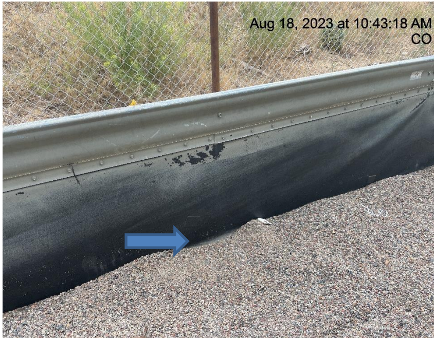
Photo # 6394 Hole in liner/liner needs maintenance
