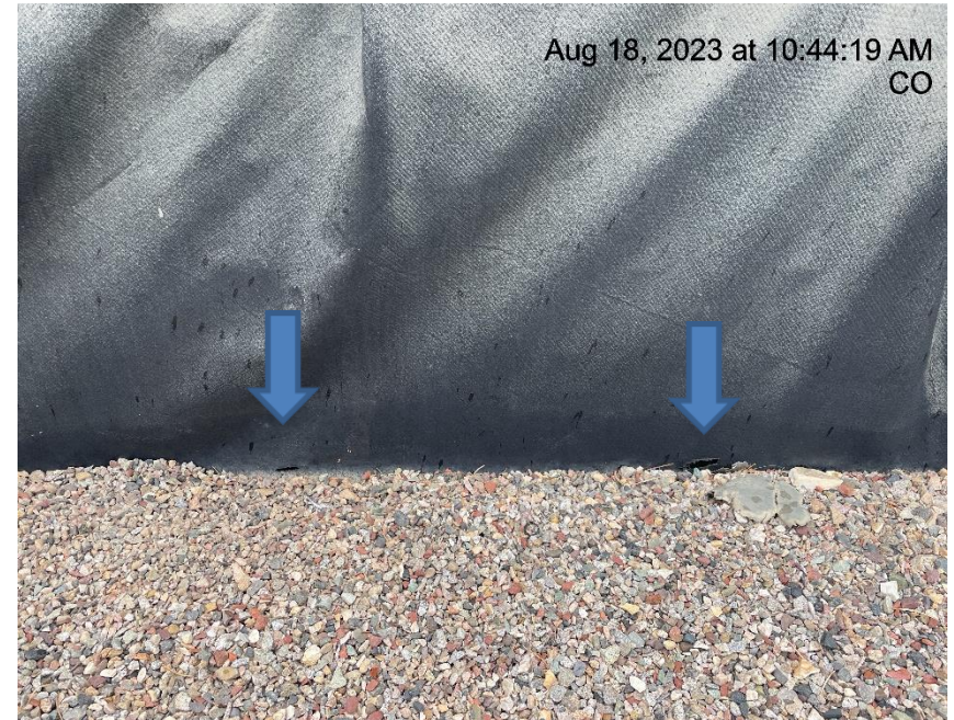
Photo # 6399 Holes in liner/liner needs maintenance
