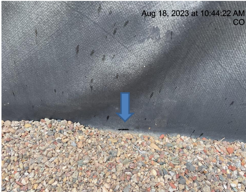
Photo # 6400 Hole in liner/liner needs maintenance
