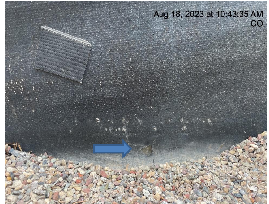
Photo # 6396 Hole in liner/liner needs maintenance
