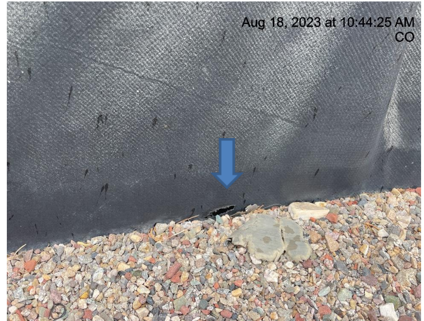
Photo # 6401 Hole in liner/liner needs maintenance
