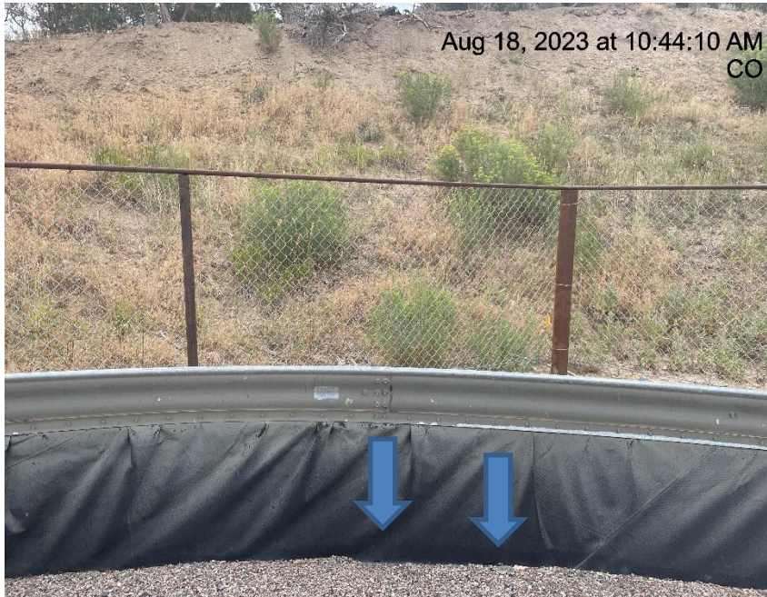
Photo # 6398 Holes in liner/liner needs maintenance
