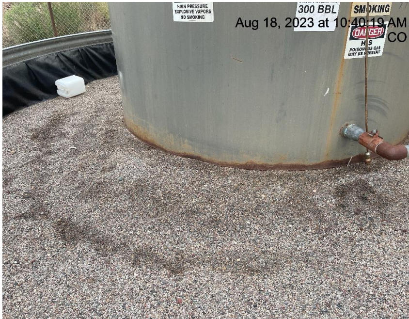
Photo # 6387 Stained gravel in secondary containment
