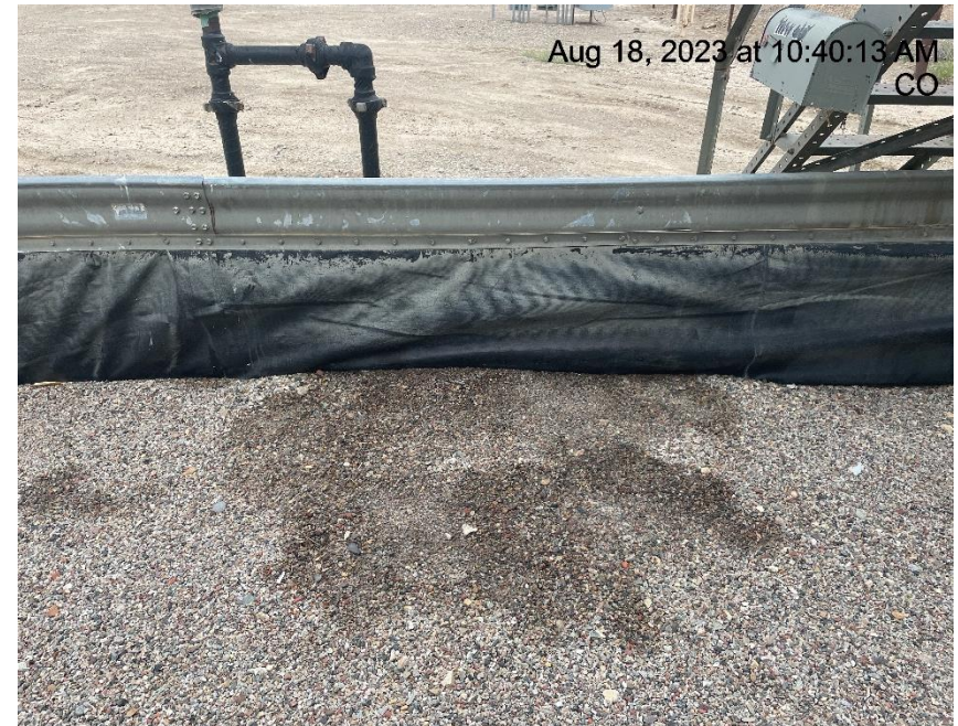
Photo # 6386 Stained gravel in secondary containment
