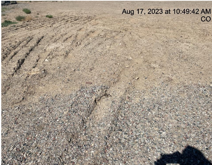
Photo # 6105 Lack of stabilization/compaction
