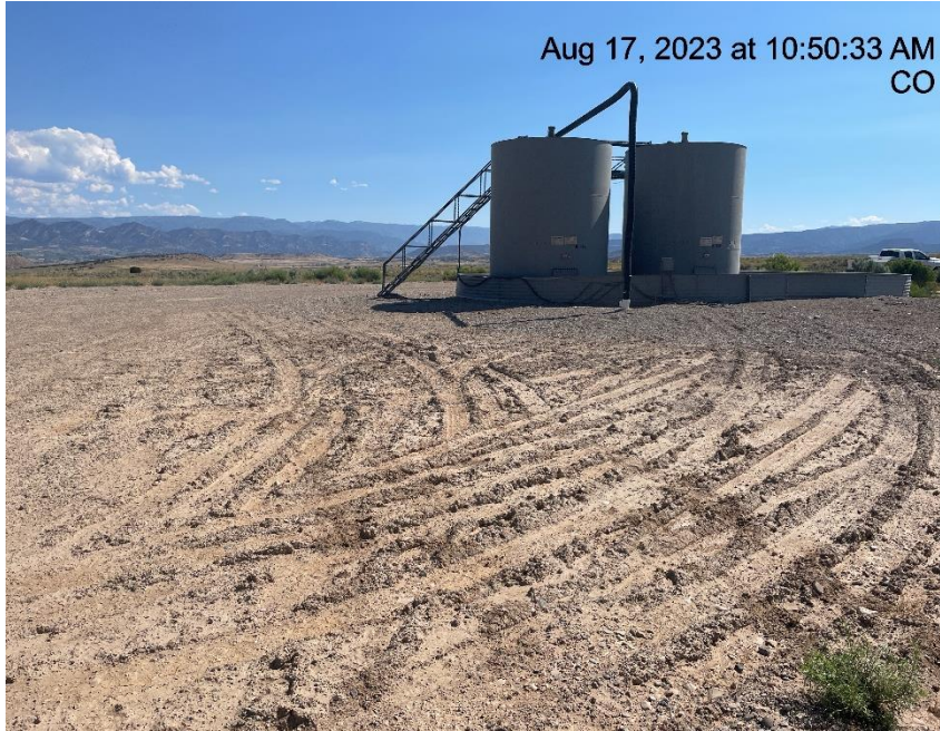
Photo # 6110 Lack of stabilization/compaction
