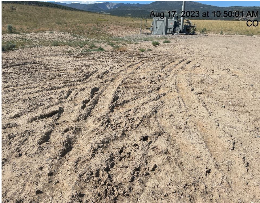
Photo # 6107 Lack of stabilization/compaction
