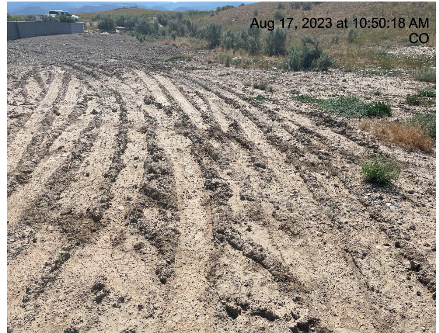
Photo # 6108 Lack of stabilization/compaction
