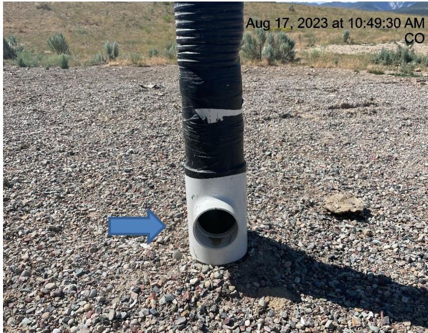
Photo # 6104 Flowline heating insulation open ended
