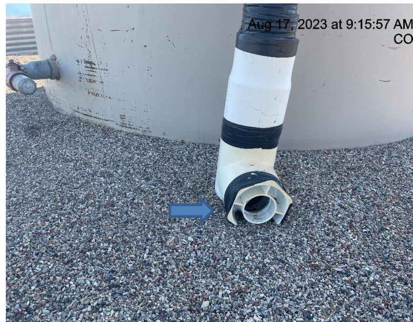
Photo # 6030 Flowline heating insulation open ended
