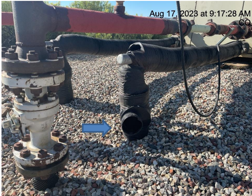
Photo # 6032 Flowline heating insulation open ended
