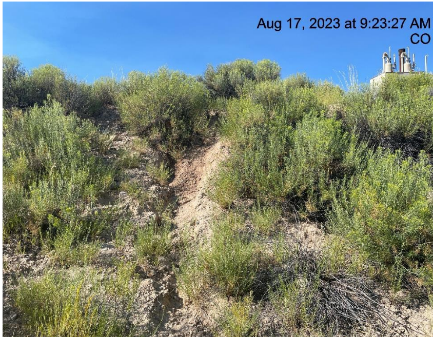
Photo # 6045 Erosion & transport of sediment off location & down slope/erosion of slope.
