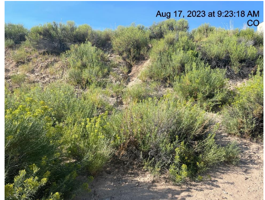
Photo # 6046 Erosion & transport of sediment off location & down slope onto another location.
