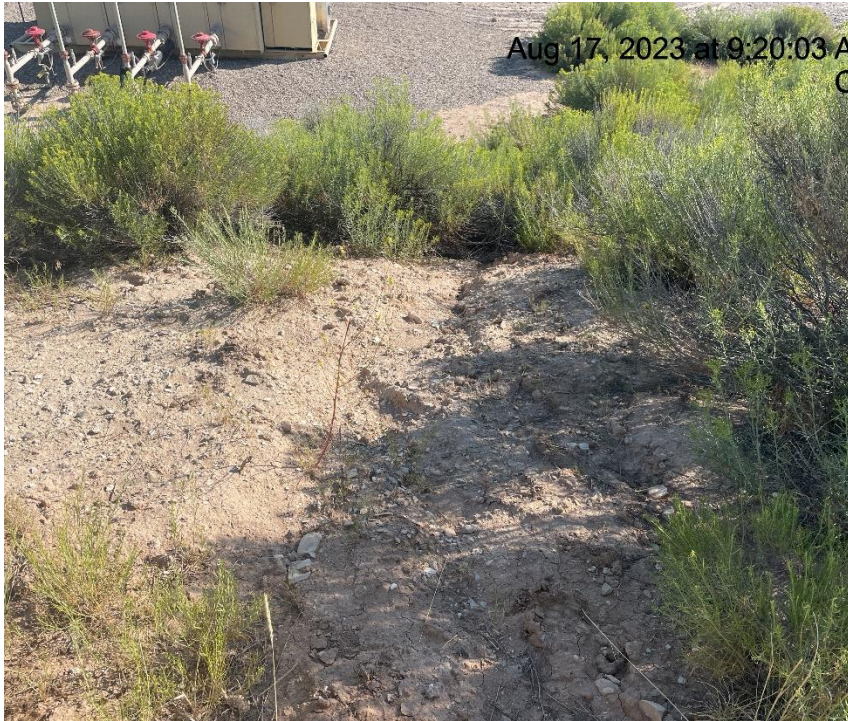
Photo # 6035 Erosion & transport of sediment off location & down slope onto another location below it.
