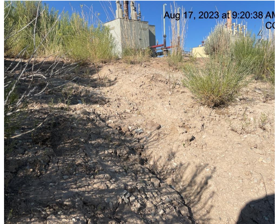
Photo # 6036 Erosion & transport of sediment off location & down slope/erosion on slope.
