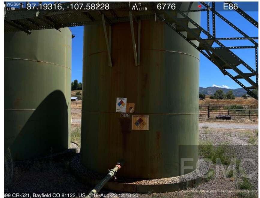
Photo #2. Produced water tank volume capacity not labeled.
