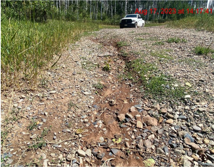
Rill Erosion on Access Road – Photo #05977
