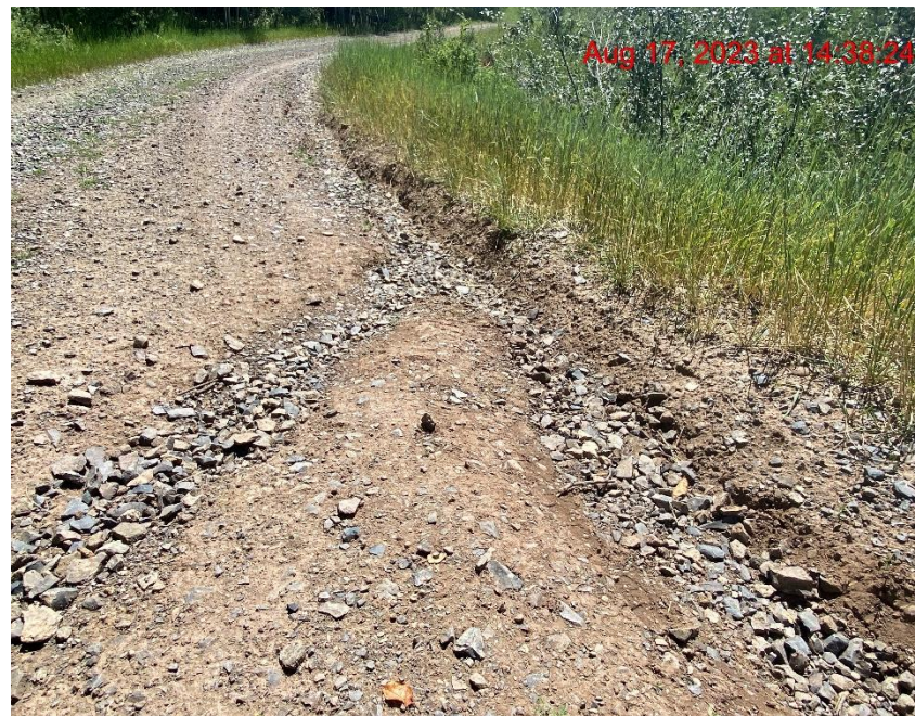
Rill Erosion on Lease Road – Photo #05981
