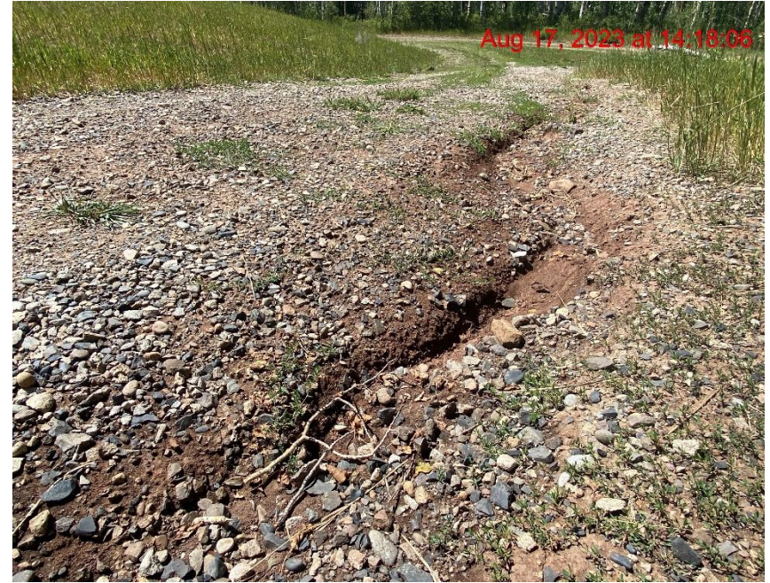
Rill Erosion on Access Road – Photo #05978
