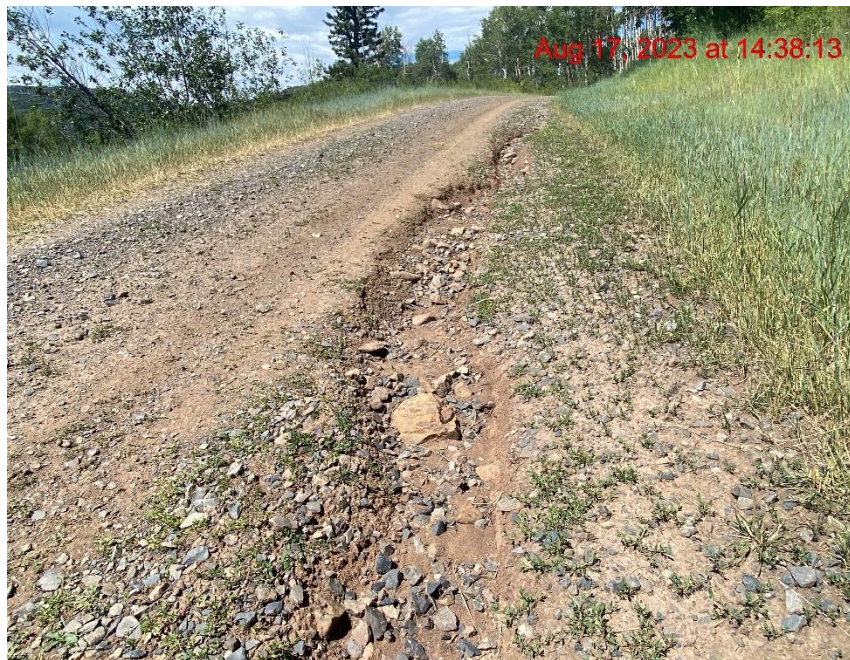
Rill Erosion on Lease Road – Photo #05980
