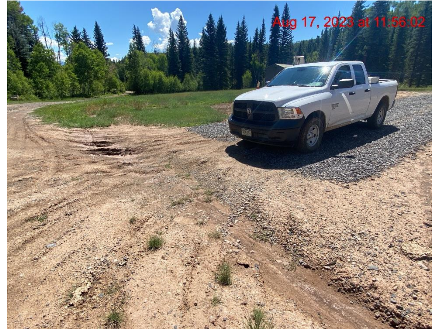
Insufficient BMPs at Ditch Crossing – Photo #05953
