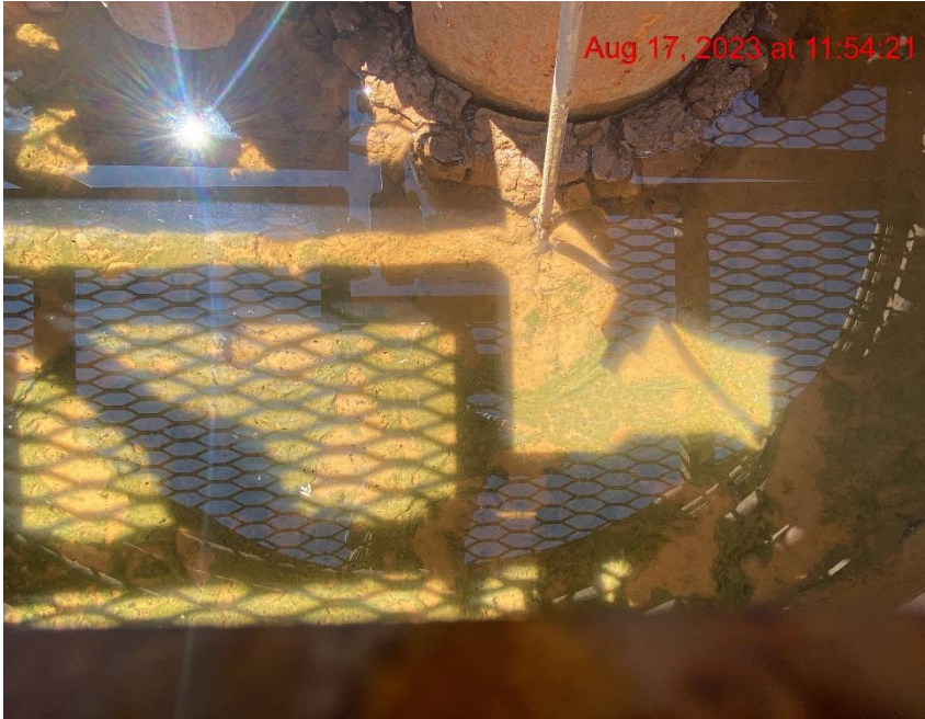
Water in Wellhead Cellar/Bradenhead Valve Not Accessible – Photo #05948
