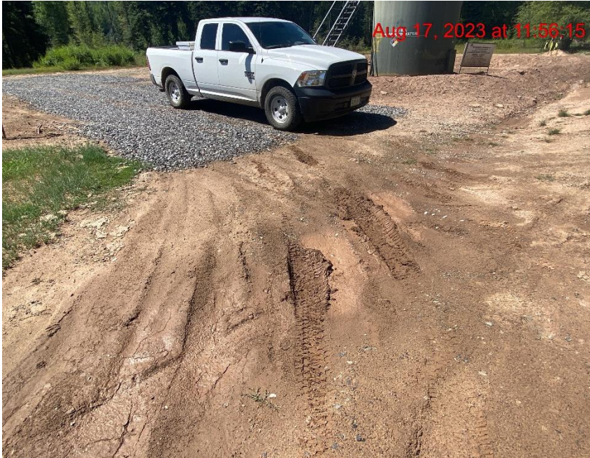
Insufficient BMPs at Ditch Crossing – Photo #05954
