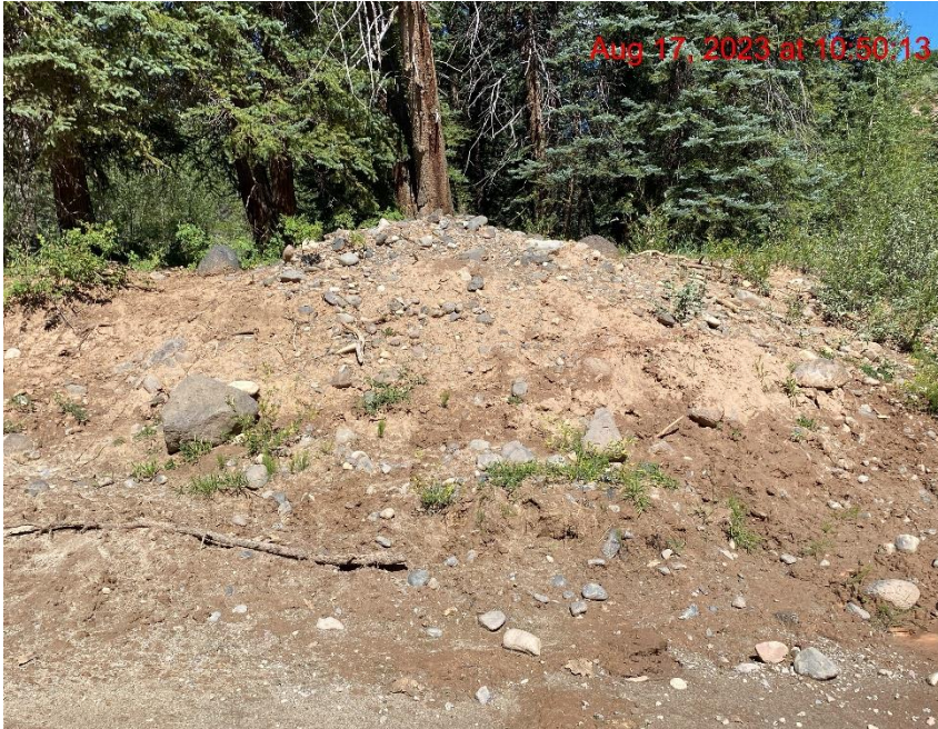
Unprotected Soil Stockpiles at Clear Fork Crossing – Photo #05920
