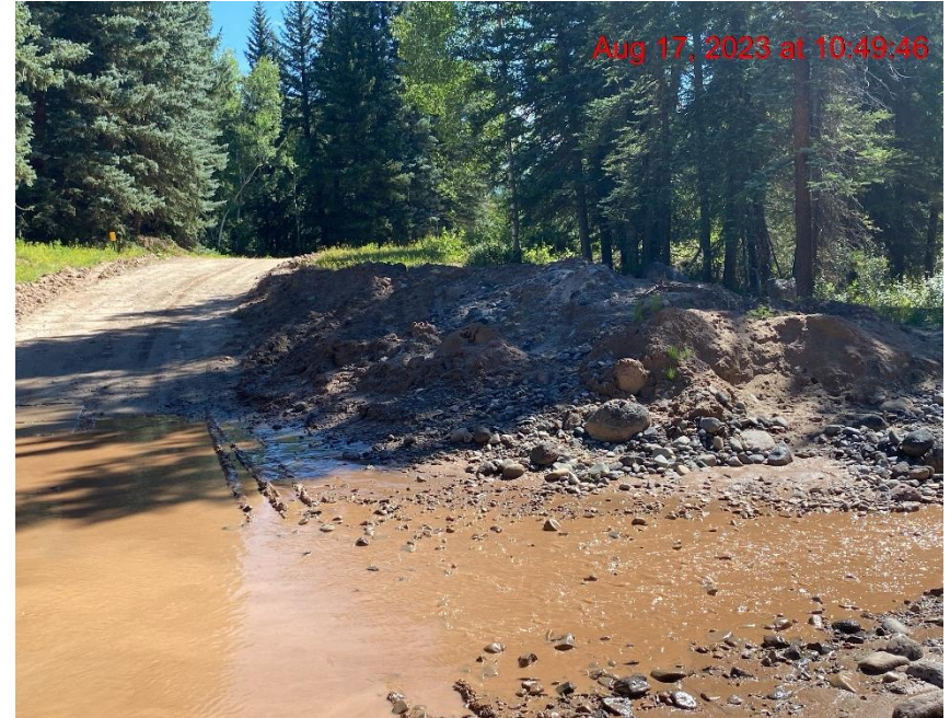
Unprotected Soil Stockpiles at Clear Fork Crossing – Photo #05917
