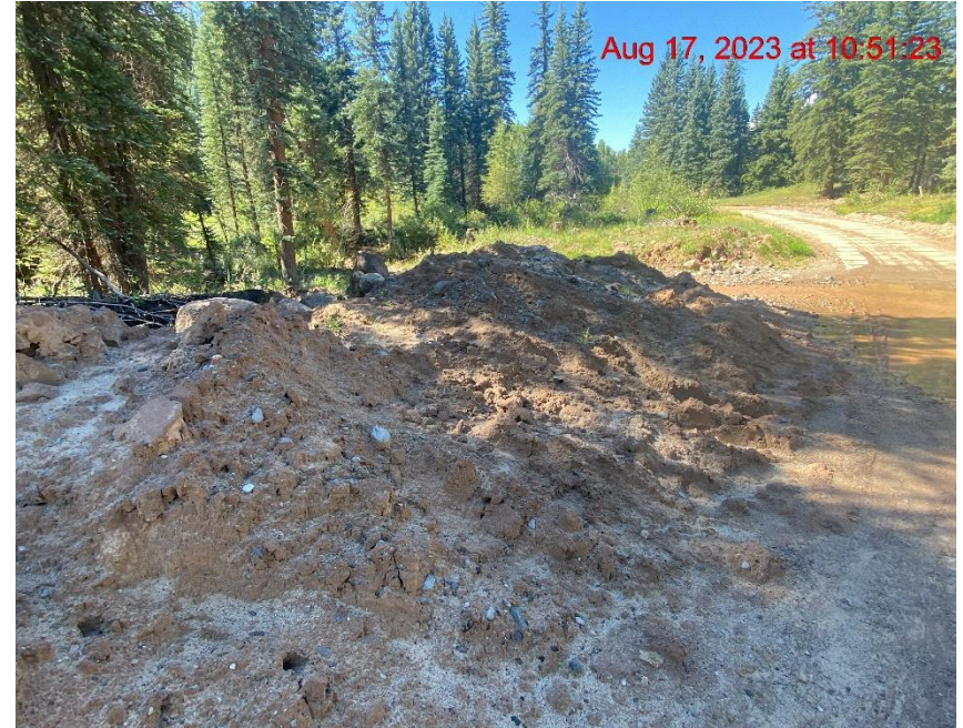
Unprotected Soil Stockpiles at Clear Fork Crossing – Photo #05921
