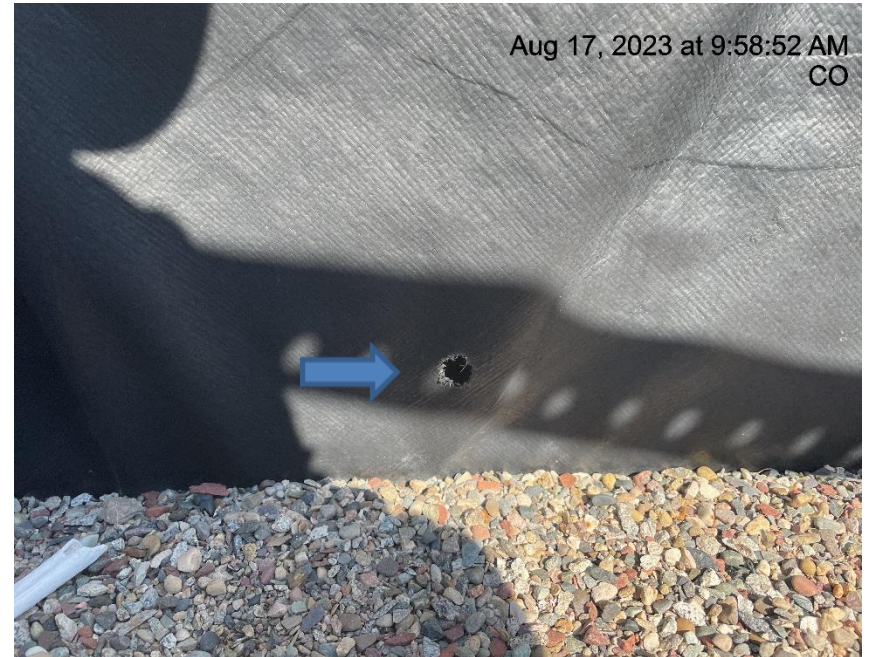
Photo # 6087 Hole in liner/liner needs maintenance
