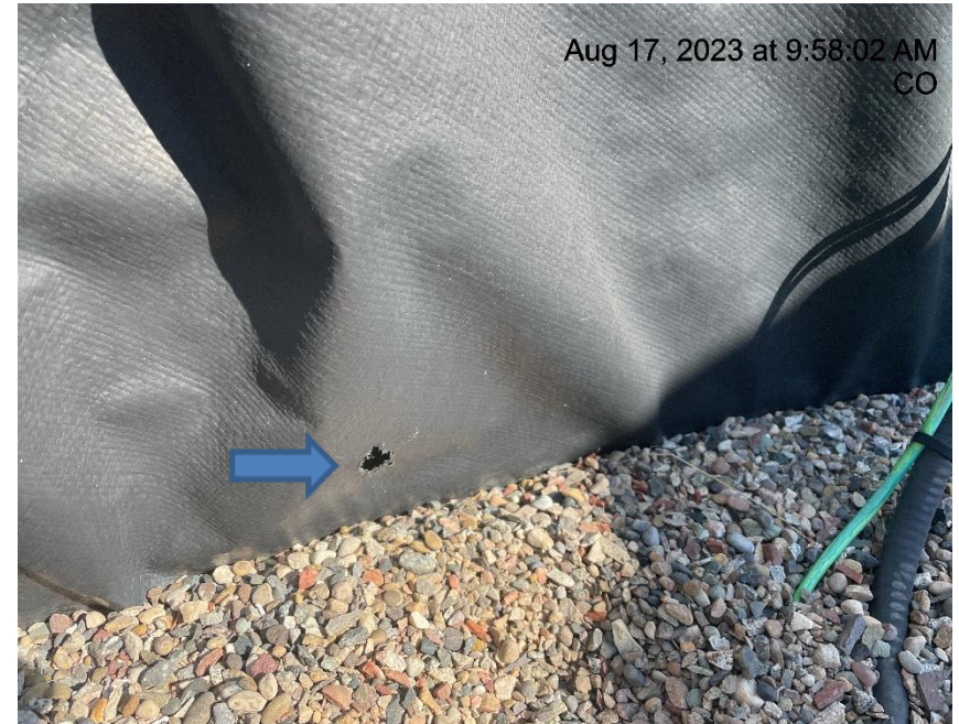
Photo # 6083 Hole in liner/liner needs maintenance
