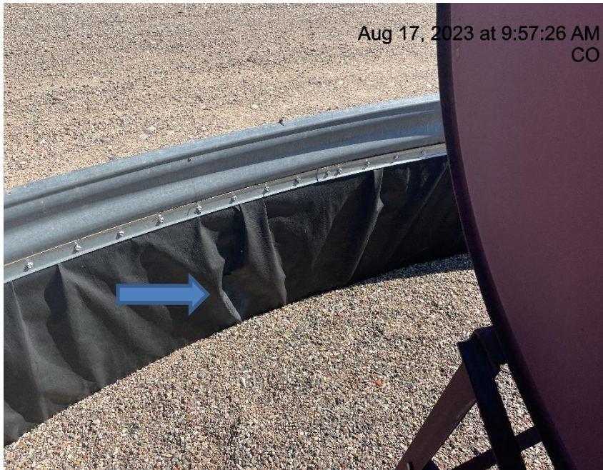
Photo # 6078 Hole in liner/liner needs maintenance
