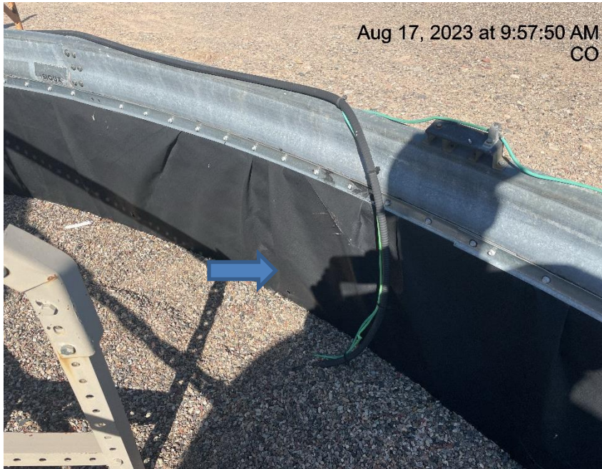
Photo # 6082 Hole in liner/liner needs maintenance
