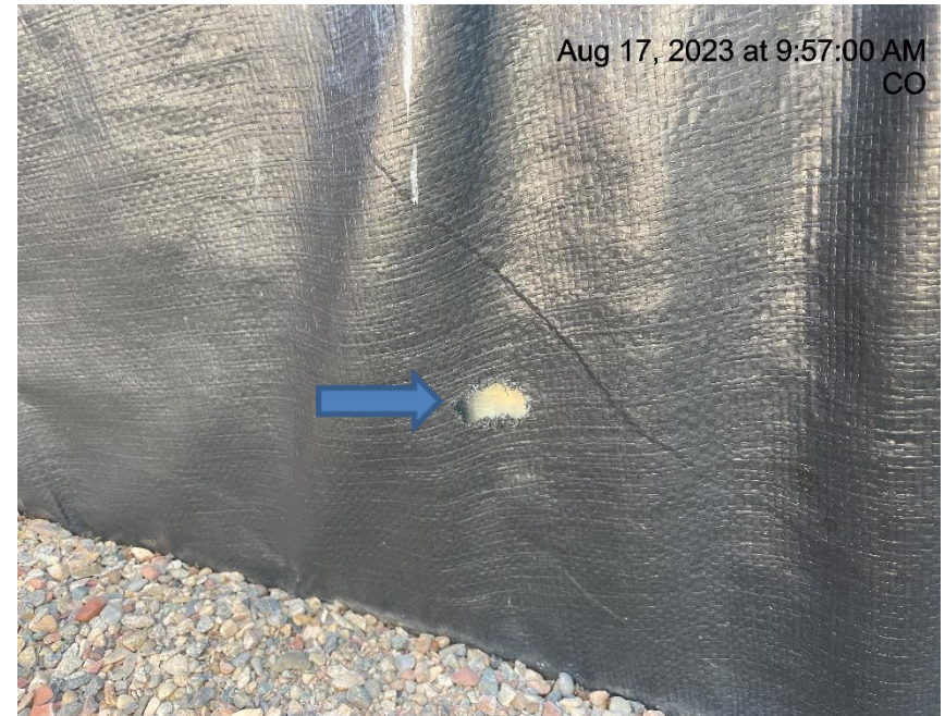
Photo # 6077 Hole in liner/liner needs maintenance
