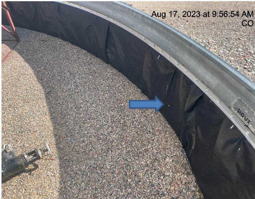
Photo # 6076 Hole in liner/liner needs maintenance
