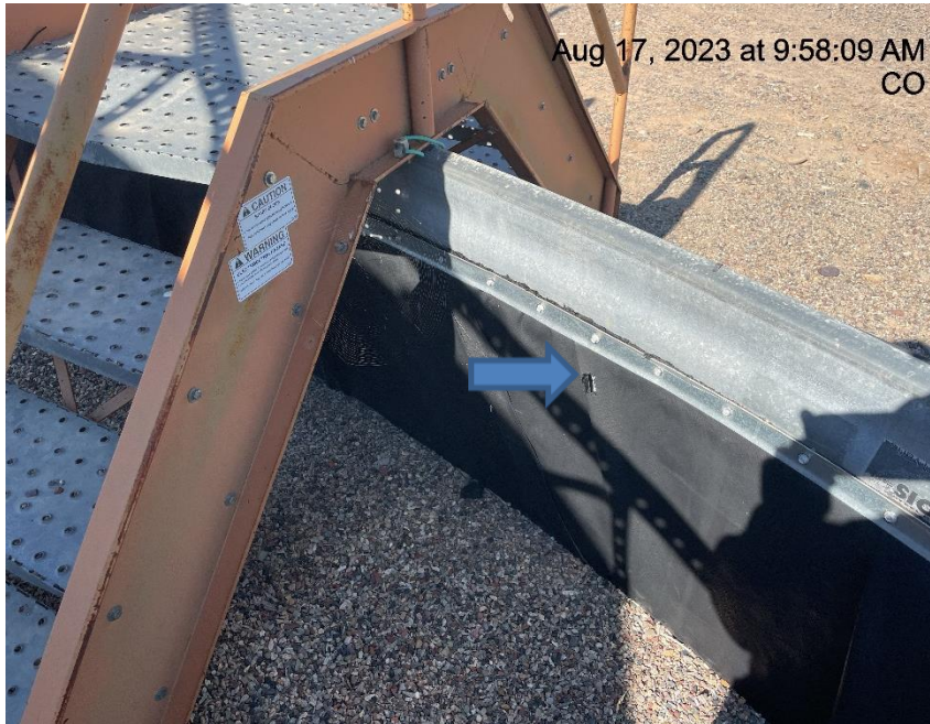
Photo # 6084 Hole in liner/liner needs maintenance
