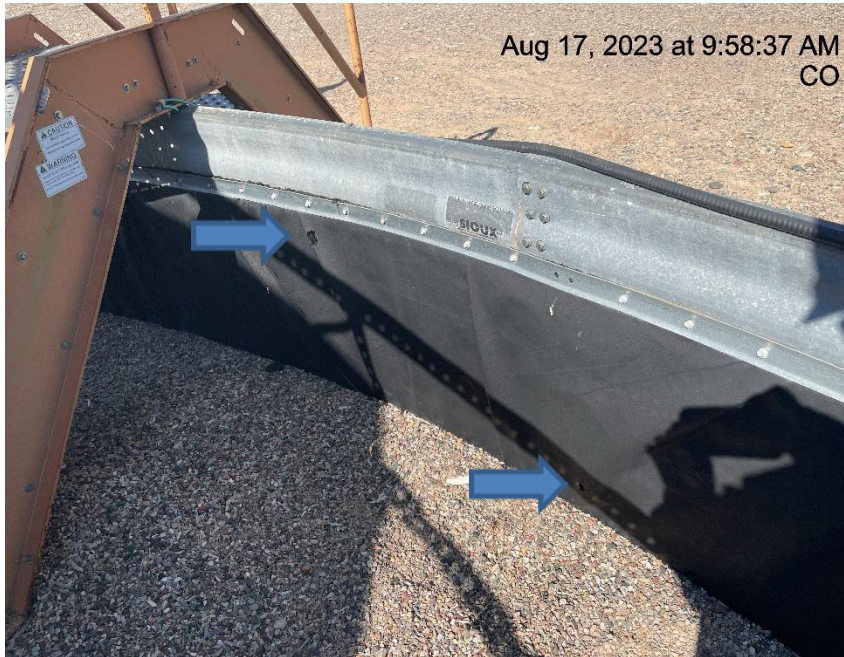
Photo # 6086 Hole in liner/liner needs maintenance
