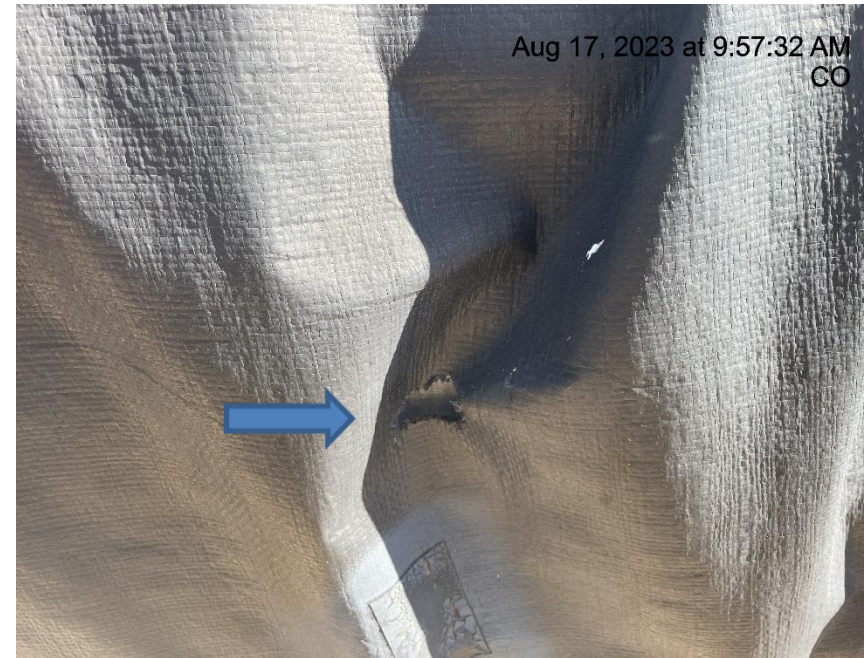
Photo # 6079 Hole in liner/liner needs maintenance
