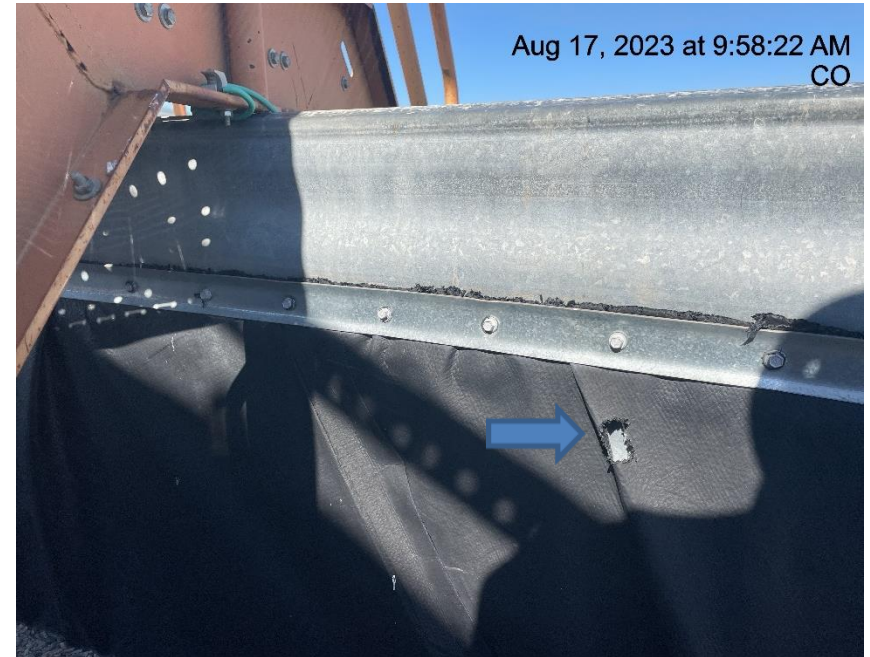
Photo # 6085 Hole in liner/liner needs maintenance
