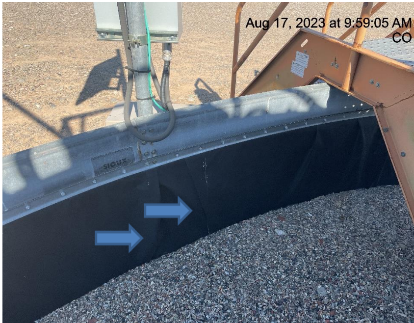
Photo # 6089 Hole in liner/liner needs maintenance
