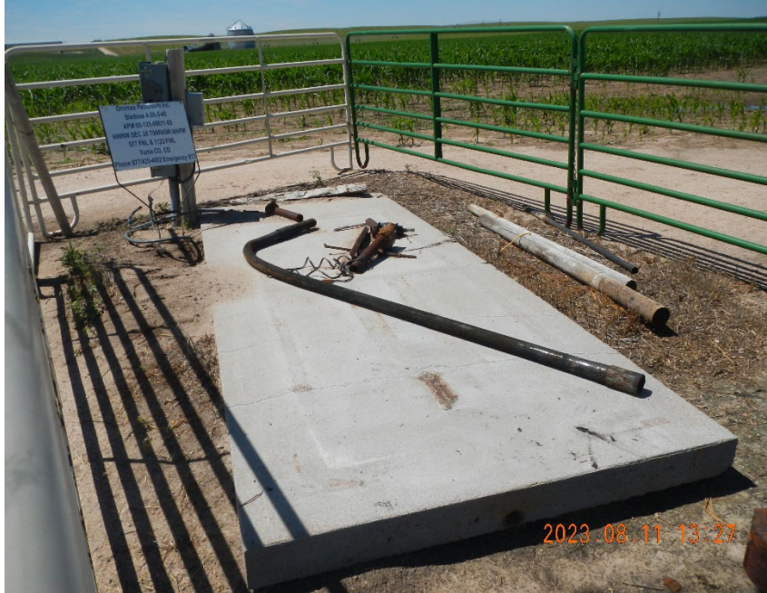
3. View of Cement Pad and production related debris. Bent tubing removed from well is laying on cement pad.
