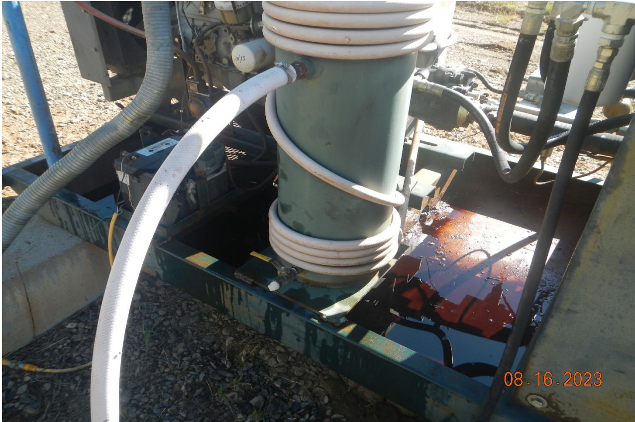
Photo 3. There are oily fluids in the engines skid that needs to be cleaned up.
