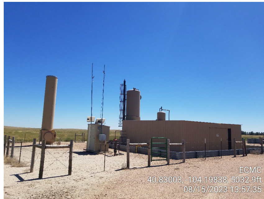
Photo 2 – Heater Treater, ECD and Gas Meter
