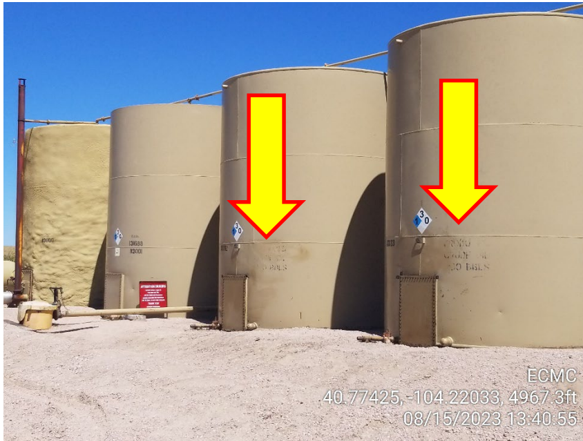
Photo 1 – Tank Battery – Labels have faded no longer visible
