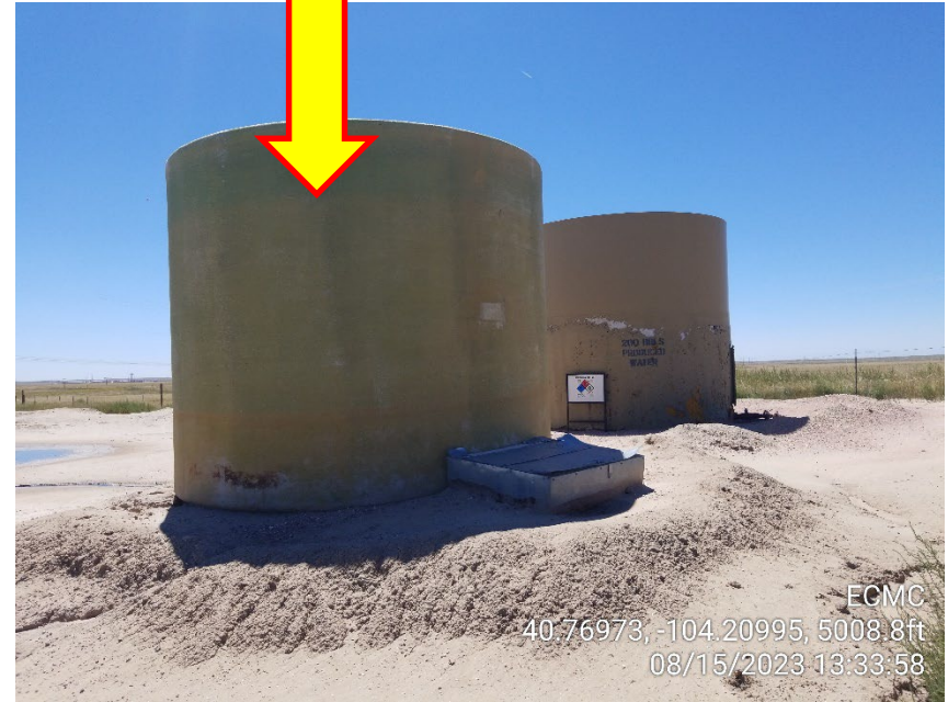
Photo 10 – Tank Labels missing
