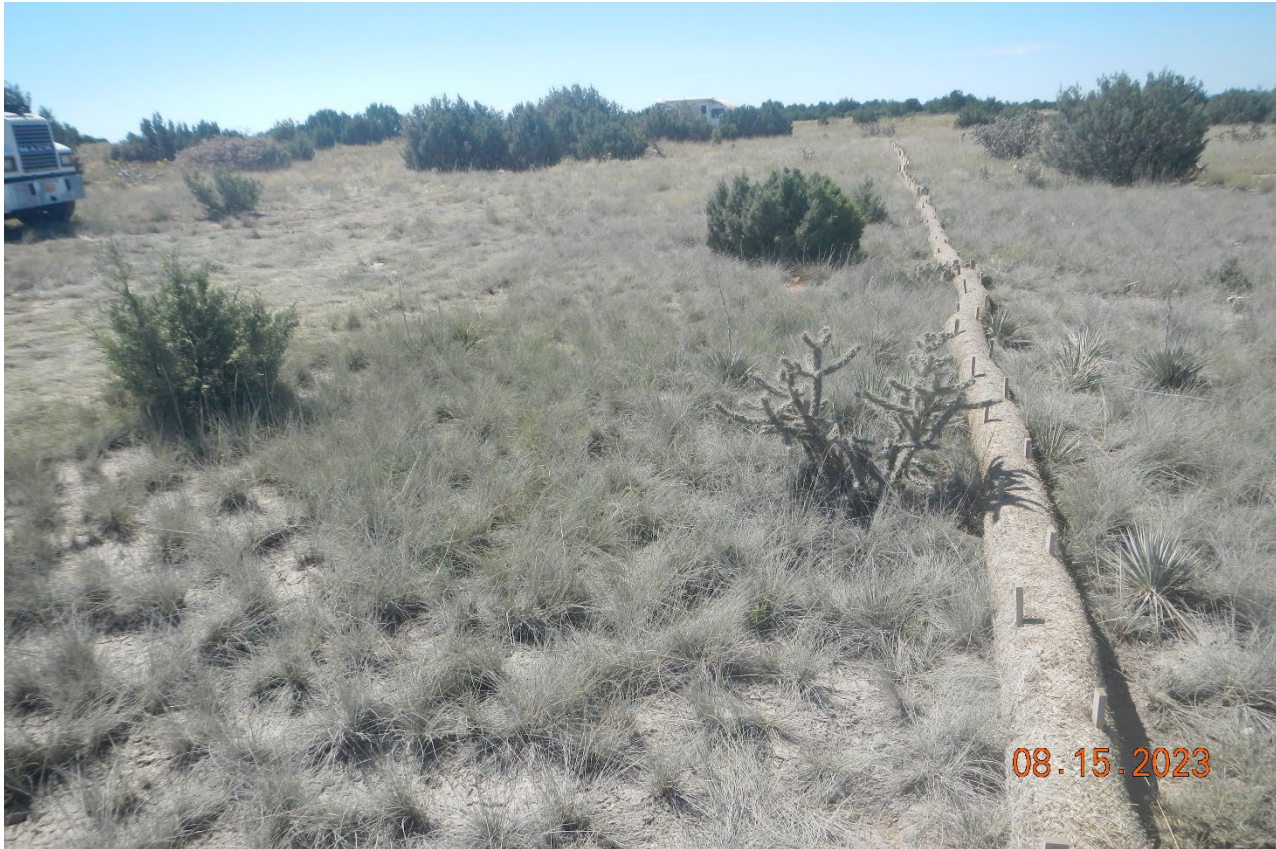
Photo 6. West side of the location facing south. Straw wattles are installed along the up and down gradient side of the location.
