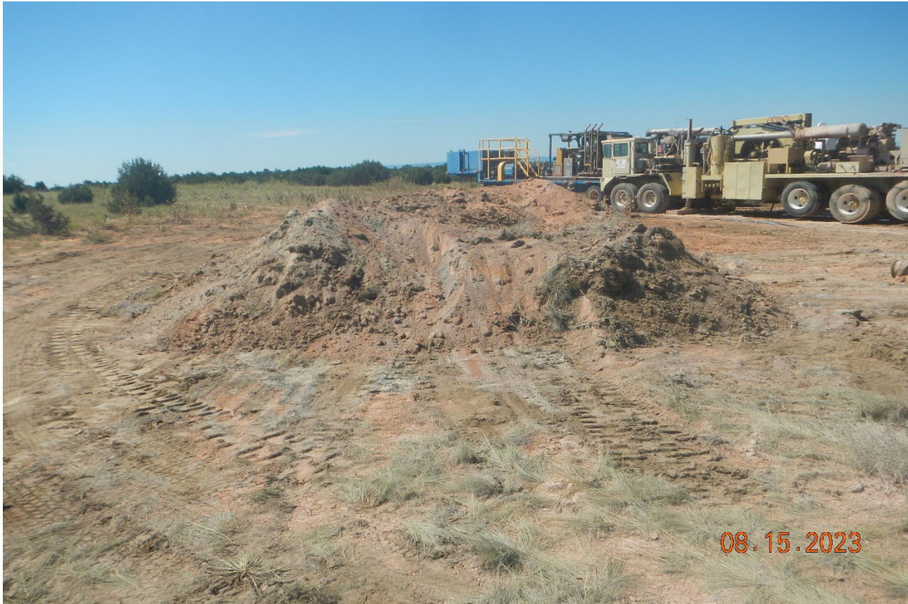
Photo 3. The cuttings pile is not stored with line and berm according to waste mng. Plan.
