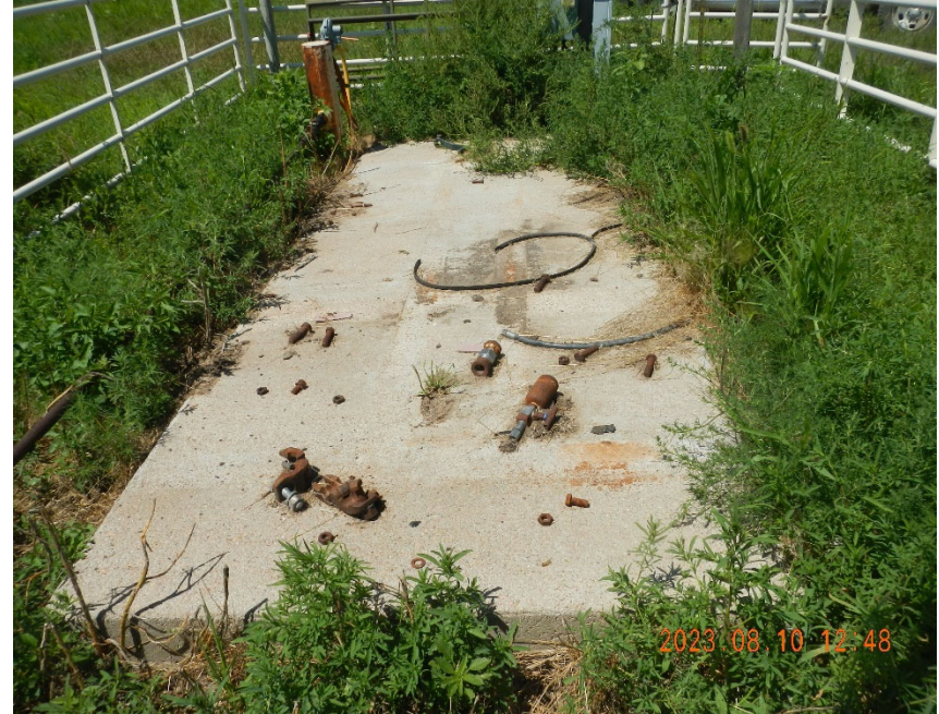
4. Cement pad left after Pump Jack removal and production related debris. Note vegetation.
