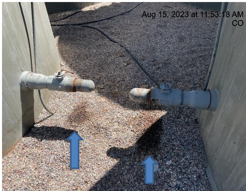
Photo # 5922 Stained gravel in secondary containment
