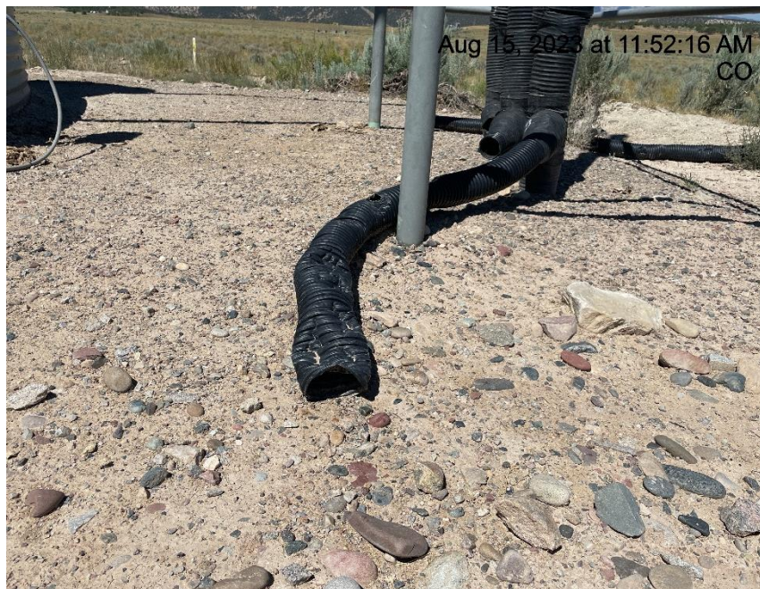
Photo # 5918 Flowline heating insulation open ended
