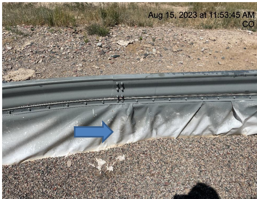
Photo # 5923 Hole in liner/liner needs maintenance
