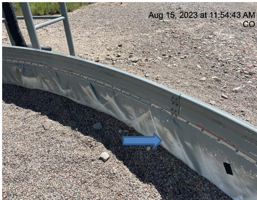
Photo # 5928 Hole in liner/liner needs maintenance
