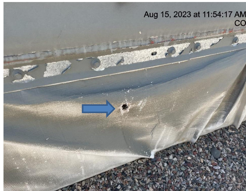
Photo # 5927 Hole in liner/liner needs maintenance
