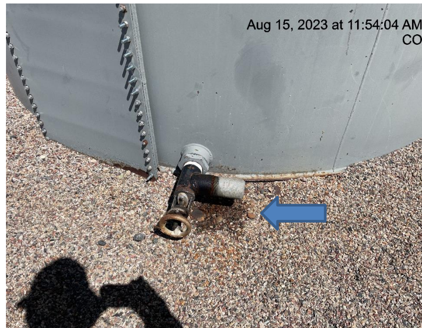
Photo # 5925 Stained gravel in secondary containment
