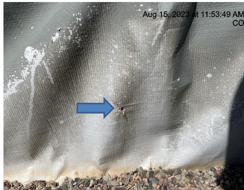
Photo # 5924 Hole in liner/liner needs maintenance
