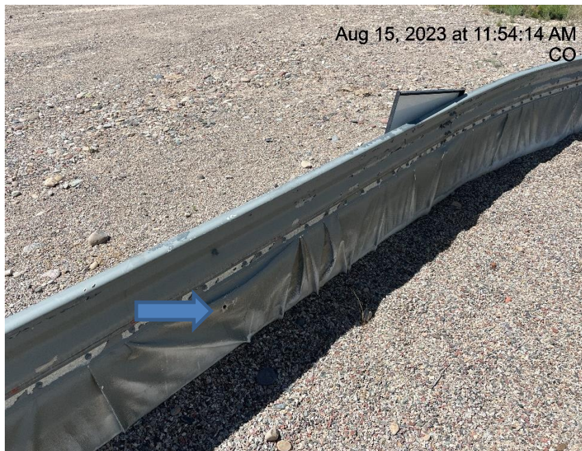
Photo # 5926 Hole in liner/liner needs maintenance
