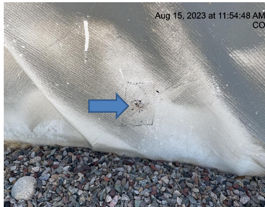
Photo # 5929 Hole in liner/liner needs maintenance
