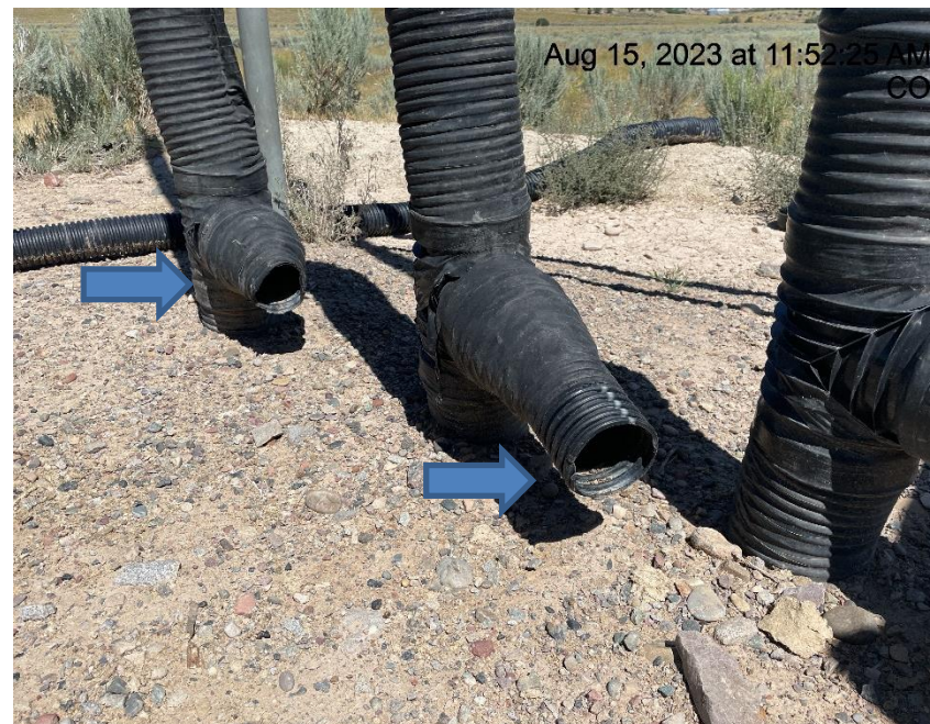
Photo # 5919 Flowline heating insulation open ended
