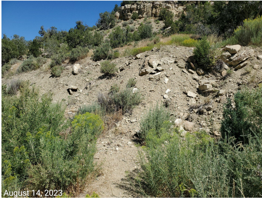
Photo 6: Unstabilized cut slopes.
