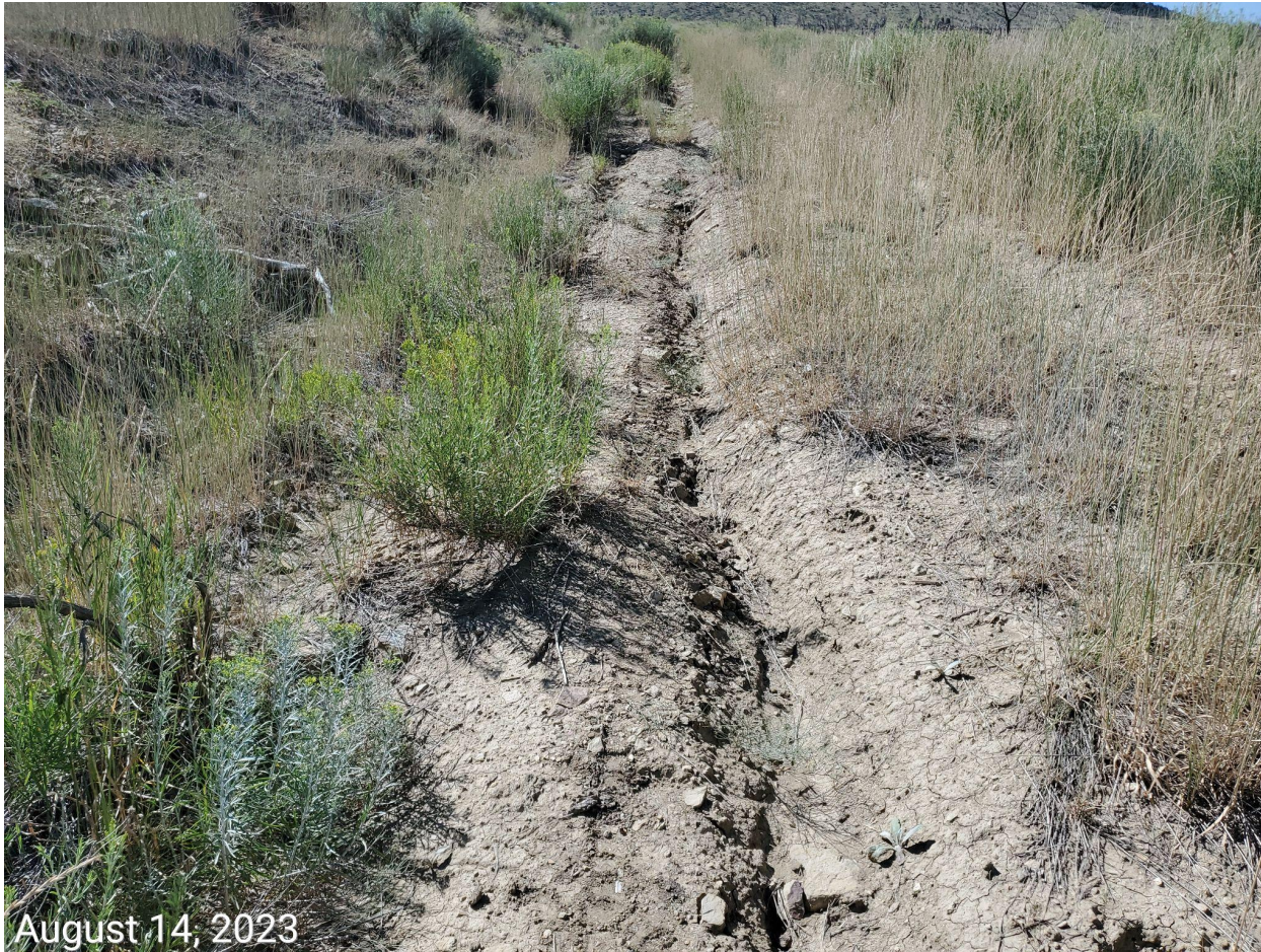
Photo 7: Photo example showing erosion degradation along access road. Stormwater and erosion control measures remain inadequate. Access road has not been decompacted, recontoured, regraded and reclaimed in accordance with 1004 Rules.
