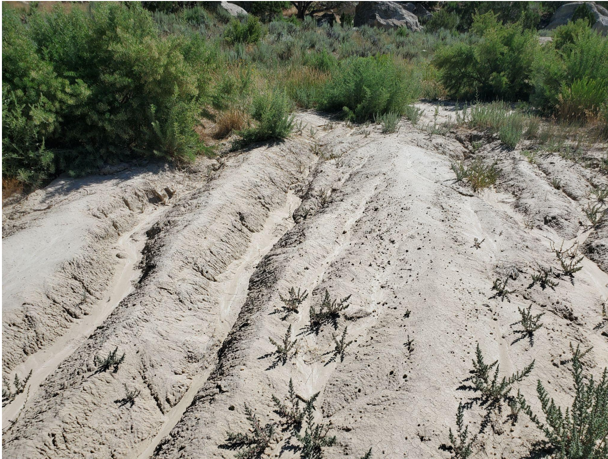
Photo 9: Photo example showing erosion degradation along access road. Stormwater and erosion control measures remain inadequate. Access road has not been decompacted, recontoured, regraded and reclaimed in accordance with 1004 Rules. Photo also shows Halogeton establishment on access road.
