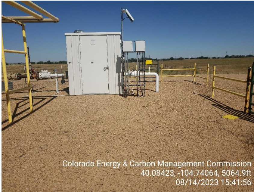
Photo 9 Gas Meter Run.
