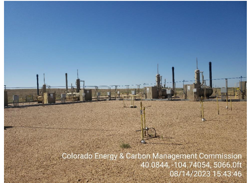
Photo 4 Horizontal heated Separators.
